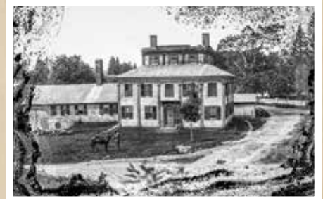
Below bottom: The Construction of Booth & Dimock Memorial Library
