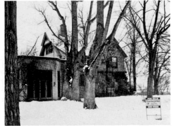
Francis G. Newlands Home, Reno, Nevada. Newlands was an influential Congressman and Senator at the turn of the century who was a strong supporter of Federal irrigation programs. He owned this large frame house from 1889 until his death in 1917. It was purchased in 1979 by the National Trust using the Endangered Properties Fund when it became known that it might be sold and either demolished or subject to intensive subdevelopment of the site. The house was in turn sold by the Trust several years later to a private owner, and preservation covenants were placed on the deed to ensure its preservation in perpetuity. Photo by Laurie Hammel.
