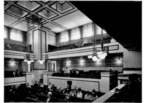
Photo of Unity Temple, Oak Park, Illinois. This architecturally significant church, designed by Frank Lloyd Wright in 1906, is one of the earliest structures that used reinforced concrete as an artistic architectural medium. It was plagued by severe roof leaks that damaged the structural and material integrity of the building until the church members and community raised private funds to make repairs. Listed as endangered in the Section 8 Report in 1983, repairs were completed in 1984. Photo by Richard Nickel.
