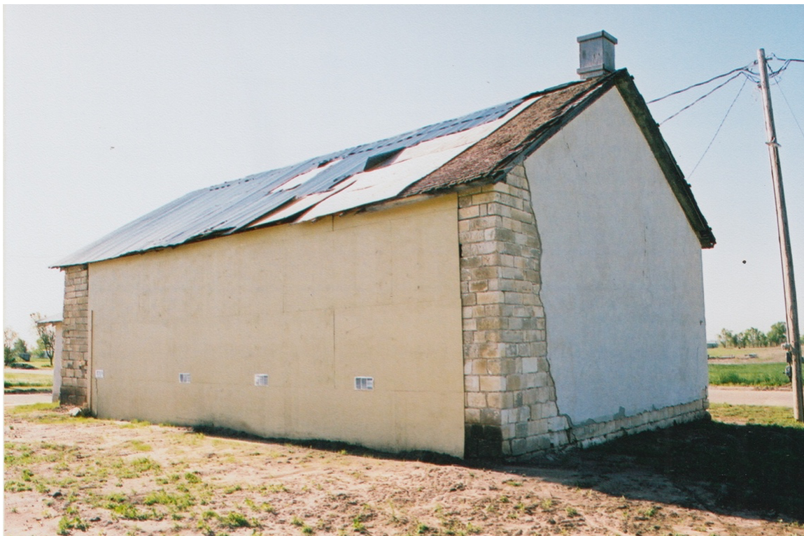
Figure 11. The AME Church in 2001, showing the temporary replacement north wall, looking southeast. Nicodemus NHS Collection, Acc no. 22, Catalog no. 20.
