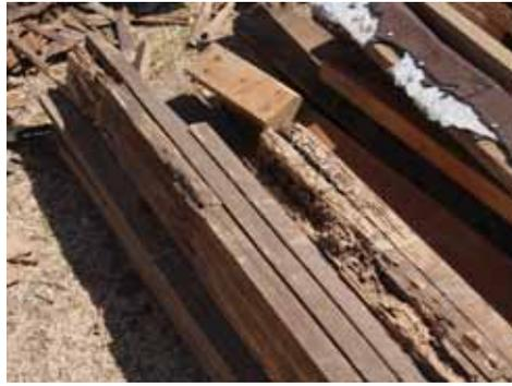
*Termite damage in some of the structural timbers that had to be replaced.*
