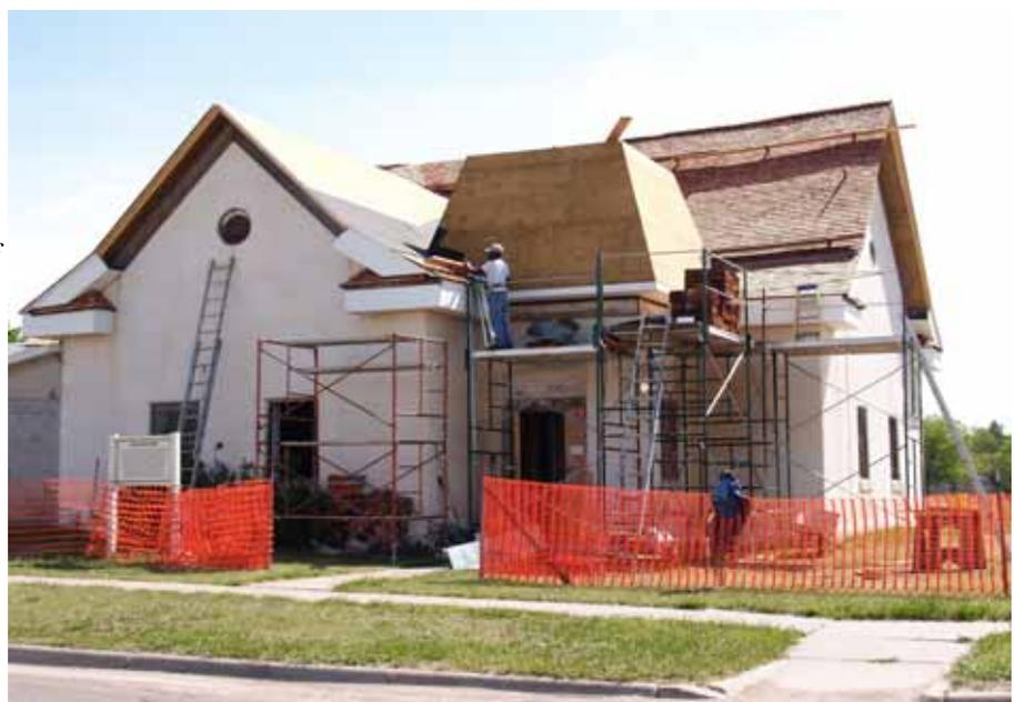
*May 16, 2006 -- All the roofing is complete, the eaves are boxed in, some of the vented window covers have been installed (to keep birds out, but let some air circulate), and shingling is starting on the bell tower. A detail photograph of the shingle pattern is included on the last page of this newsletter. (All Photos: NPS)*
