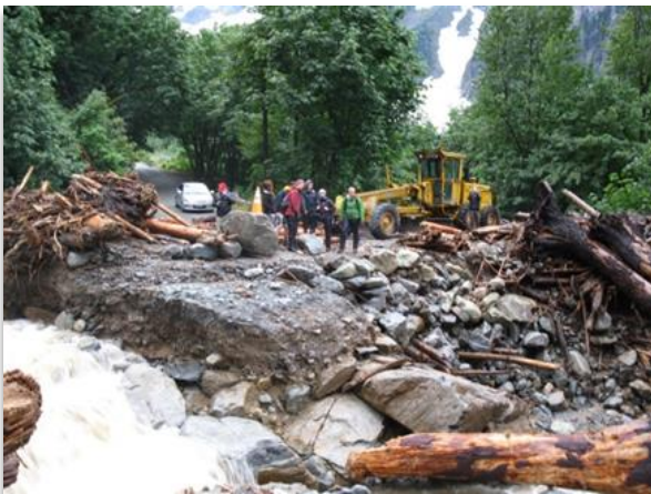
Figure 3. Cascade River Road, August 2013. Heavy rain mobilized river debris clogging a culvert. The road washed out, stranding 70 visitors and their vehicles for 2 days.
