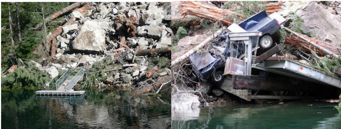
Photo 2. Debris avalanche in 2013 just below Ross Powerhouse in Skagit Gorge.
