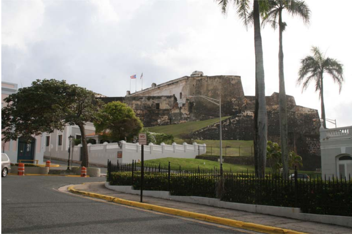
Castillo de San Cristóbal and Casino de Puerto Rico (right), camera facing northeast (above).
