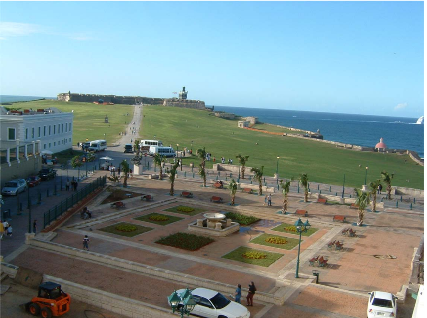
Jardín de Ballajá (foreground), Asilo de Beneficencia, Asilo de Locos, Morro Esplanade, and Castillo del Morro (background), camera facing northwest. Photograph by OECH, 2003.
