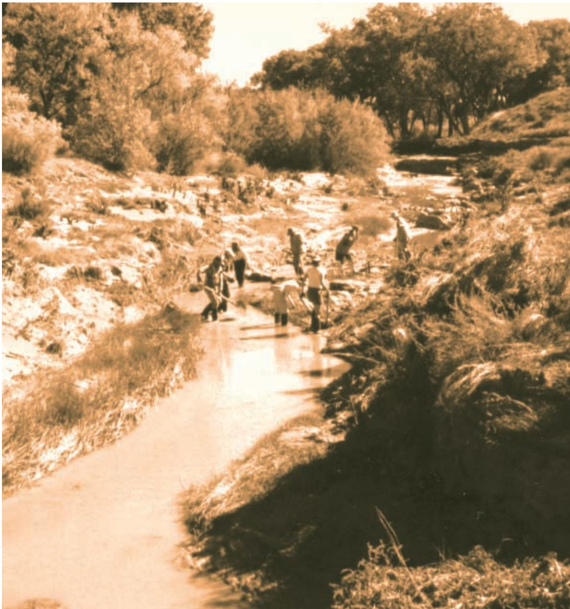
Volunteers construct small water-diversion structures within Pueblo Colorado Wash to encourage the formation of stream meanders. The work is part of a three-year demonstration restoration project at Hubbell Trading Post National Historic Site.
