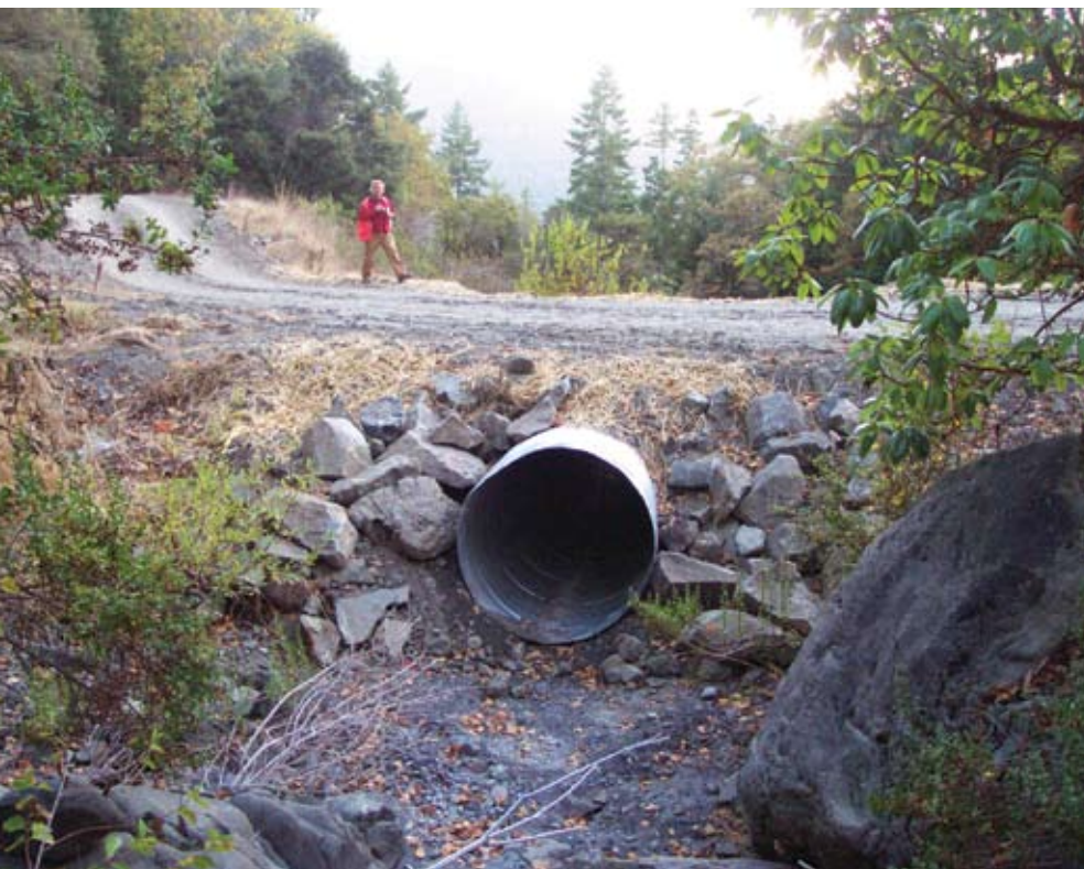
During restoration of Coyote Creek basin, the National Park Service and its cooperators installed new, larger-diameter culverts at stream crossings. The old culvert at this crossing was severely rusted and substantially undersized for even moderate winter storm flows. The new culvert is 60 inches (150 cm) in diameter, which is large enough to accommodate a 100-year flood.
