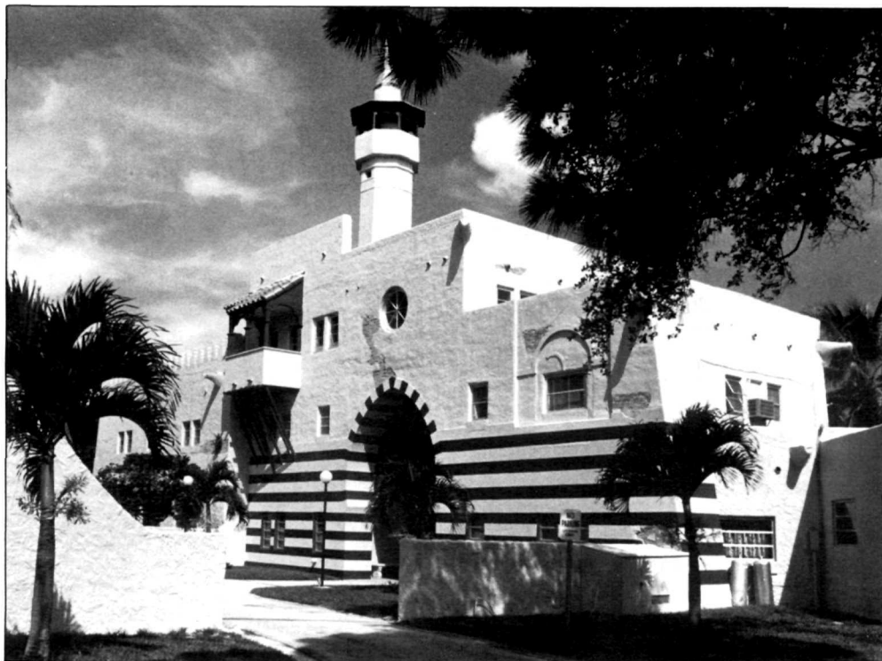
Opa-Locka Company Administration Building, Opa-Locka, Florida: anchor building for planned city conceived by inventor and real estate developer Glenn Hammond Curtiss (Mary Evans).
