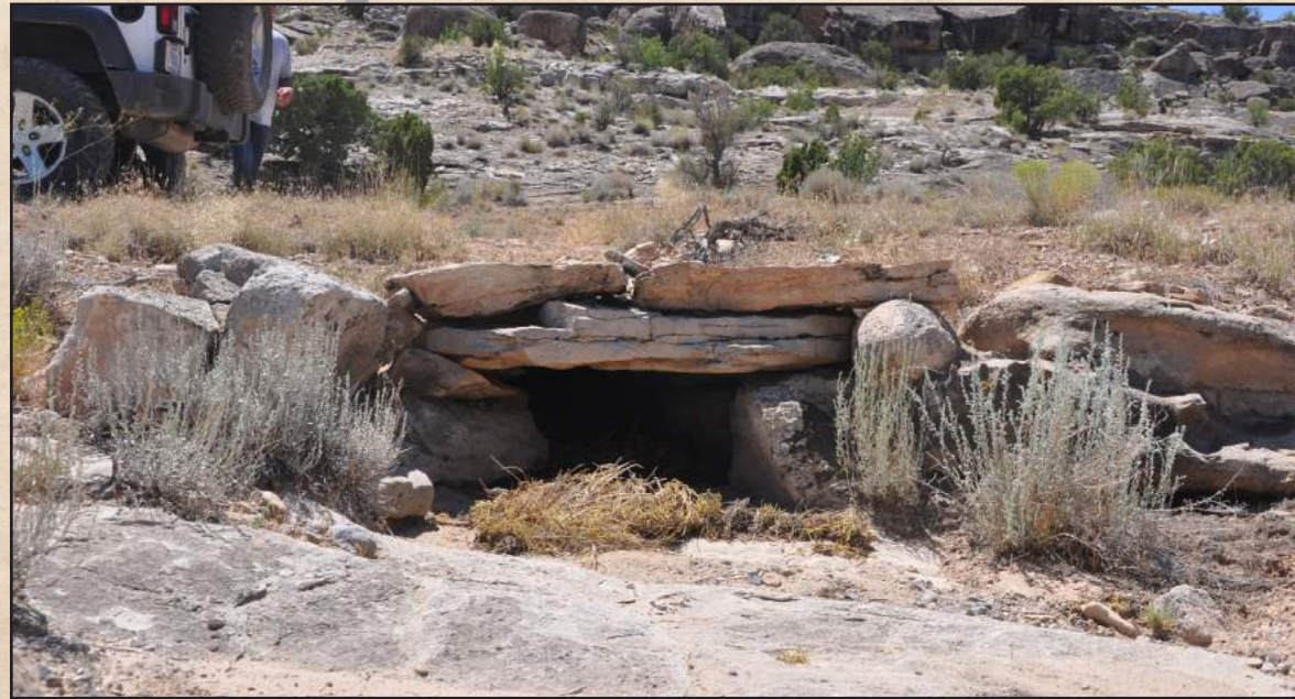
Culvert on Lost Springs Road
