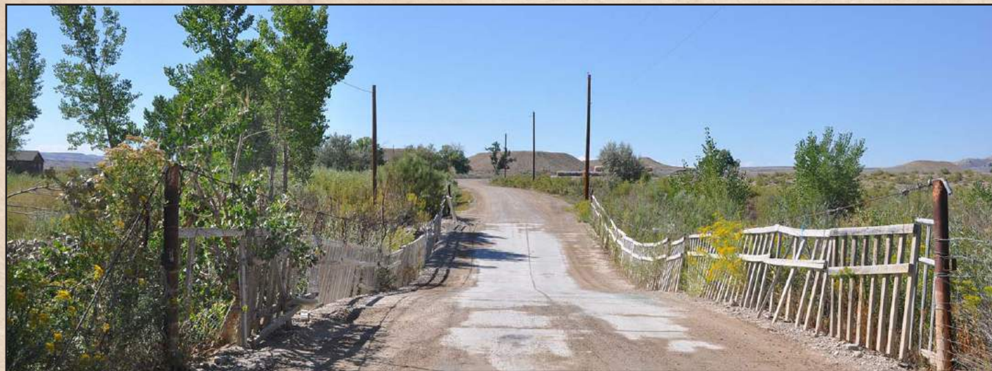
Bridge over Ferron Creek outside of Ferron, Utah
