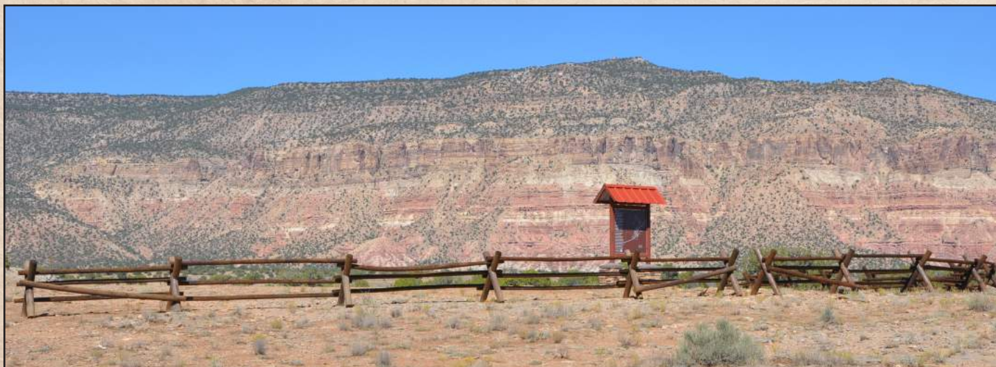
Spirit Railroad Complex kiosk and rail fencing
