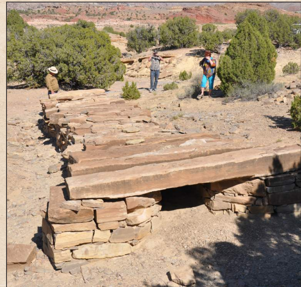
Exposed stone culvert
