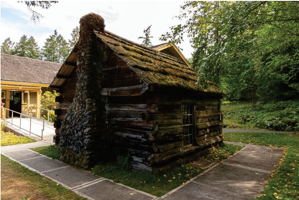
Figure 4 of 5. Corner view of the west and south elevations of Beaumont Cabin, facing east.
