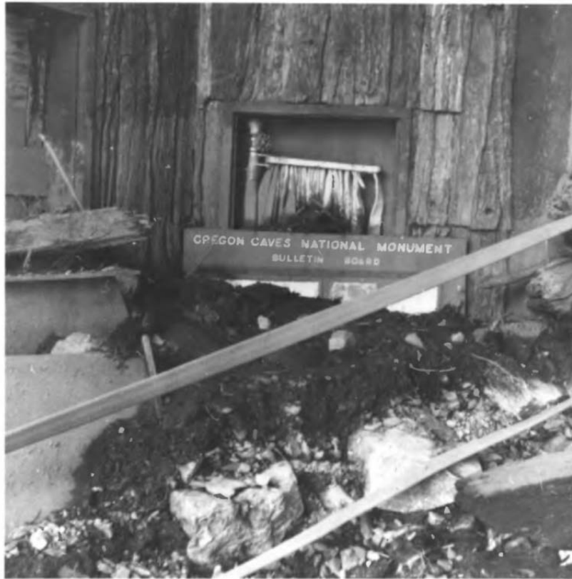
Figure 7. Mass-wasting hazard. In December 1964, a debris flow entered the Chalet and deposited an estimated 2,600 m 3 (3,400 yd 3 ) of material in the breezeway. National Park Service photograph, printed in Friday (1983).
