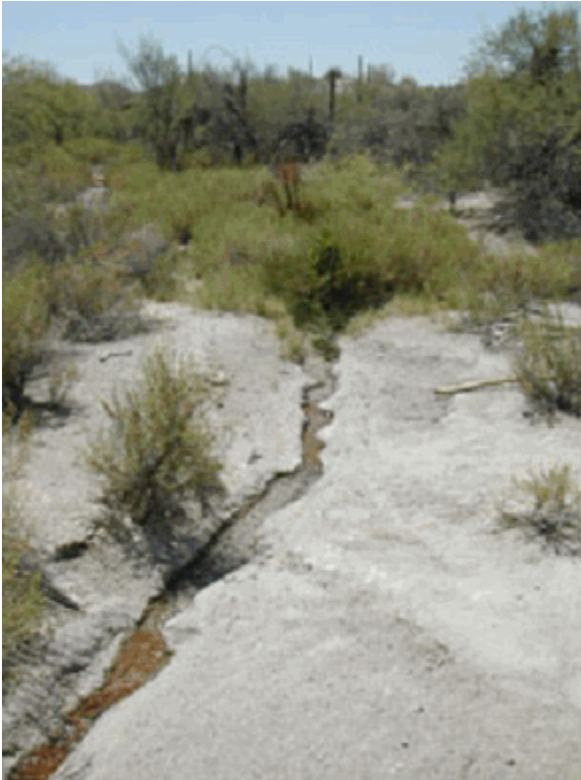
Concrete channel constructed in 1989 to direct water from springs to pond (Photo by J. Galbraith, 2002)
