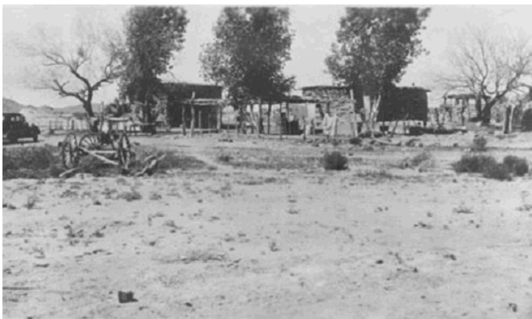
Corrals and buildings used by the Orozco family at Quitobaquito. Structures were razed after 1957 (Photo by N. Dodge, F. Pinkley, J. Miller, May, 1939) ORPI#507)
