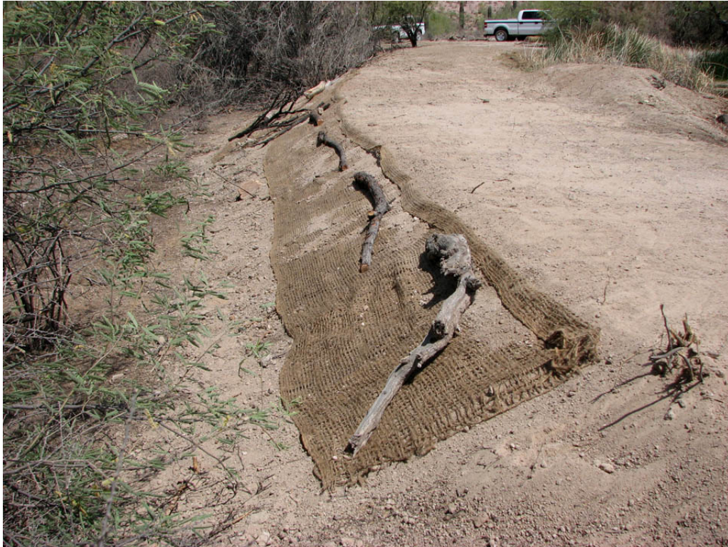
Figure 15. Jute erosion matting and mesquite branches placed to minimize erosion on outside face of the retaining berm. View is to northwest. Quitobaquito Pond, Organ Pipe Cactus National Monument, Arizona.
