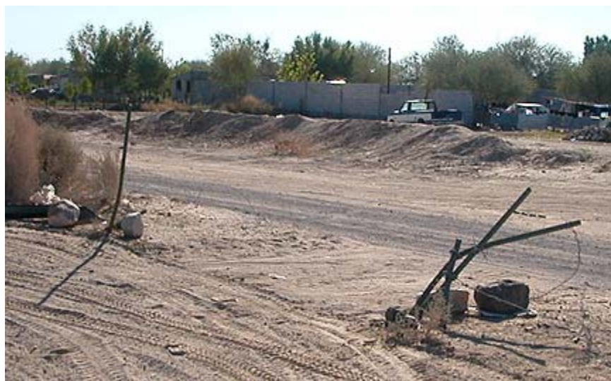
Figure 13: Existing Breached Border Fence
