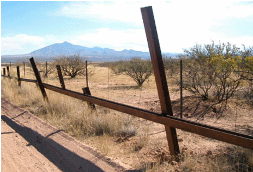
Figure 3: Existing Vehicle Barrier East of Coronado
