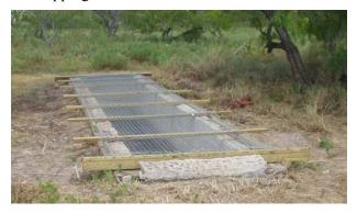
made depression. Mesquite trees and undergrowth such as grasses, shrubs, and prickly pear cacti surround the area. The tank is rectangular, bricklined, approximately 6' x 35', and is below grade. The man-made depression is approximately 5' x 25' and was likely used to dump spent solution or clean-out sludge from the tank. The cattle dip tank has been secured to prevent access. An asphalt walkway, heading from the park's visitor's center, is located about 200-feet south of the dipping tank area.
