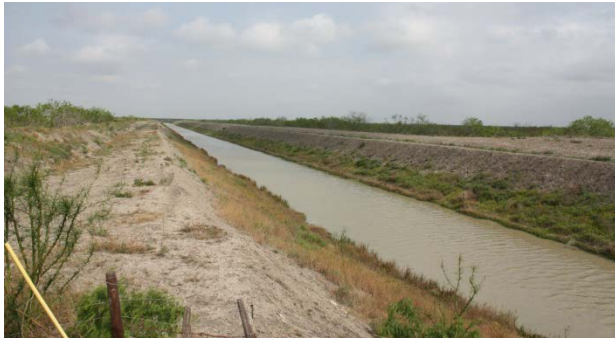
Figure 10. Photograph of canal. The canal along the northern boundary of the park was constructed in 1916 for flood control and drainage. The canal excavation reaches approximately 9 m (30 ft) below grade. National Park Service photograph by Rolando Garza (Palo Alto Battlefield NHP).
