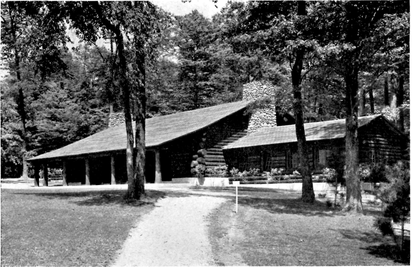
Administration Building, Selkirk Shores State Park, New York
