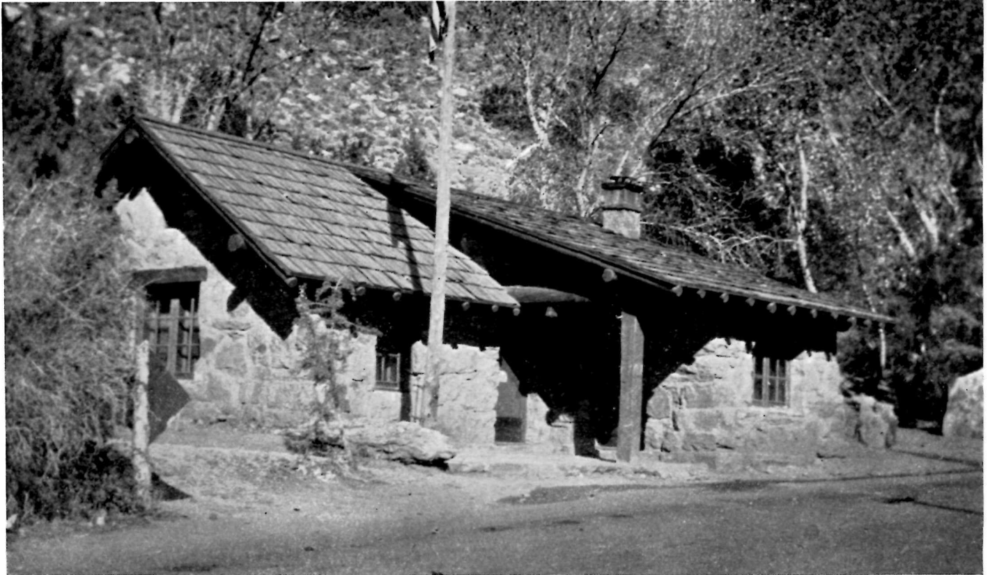
Administration Building, Zion National Park
