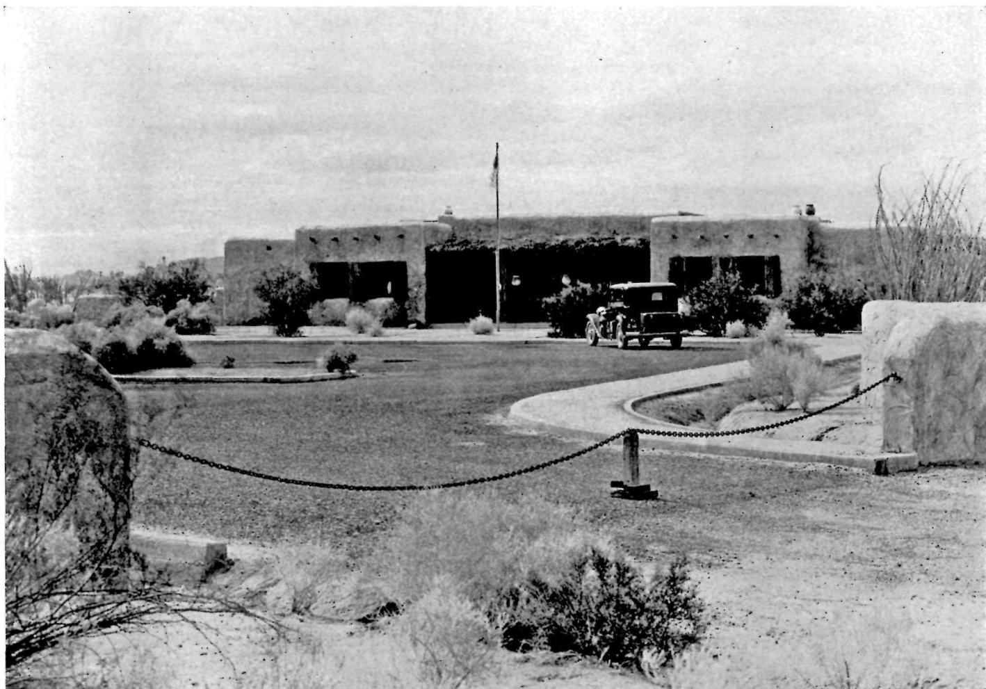
Administration Building, Casa Grande National Monument
