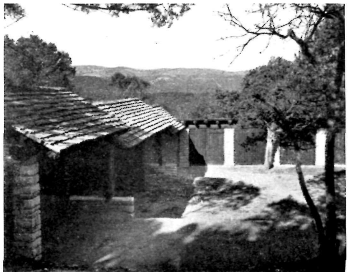
Service Group, Garner State Park, Texas
