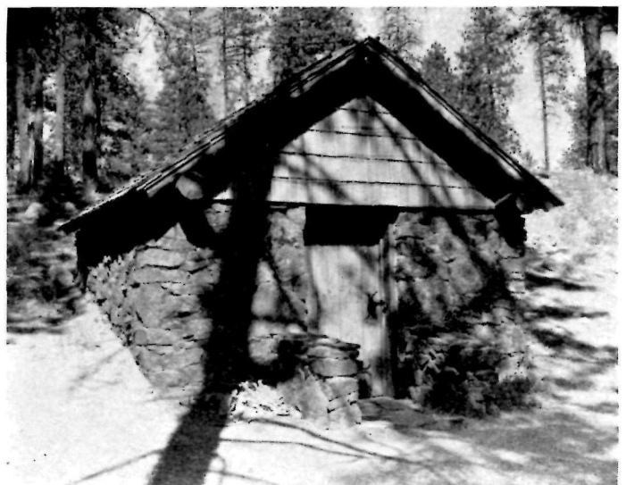
Utility Building, Riverside State Park, Washington
