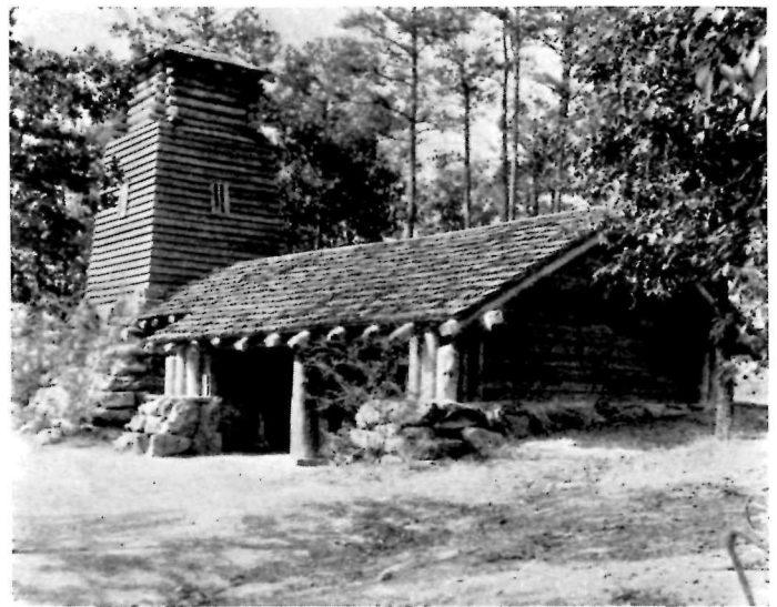
Custodian's Garage, Boyle Metropolitan Park, Little Rock, Arkansas
