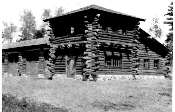
Equipment Building, Itasca State Park, Minnesota
