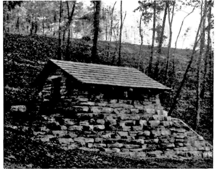
Pumphouse, Devil's Den State Park, Arkansas
