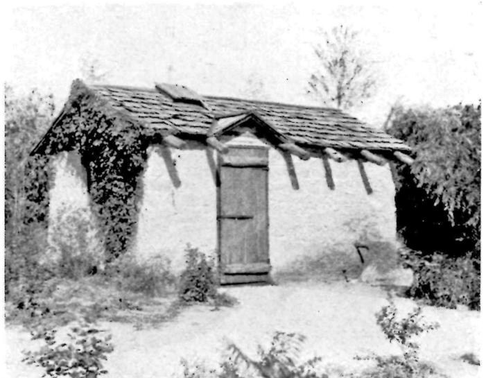
Pumphouse, Pere Marquette State Park, Illinois
