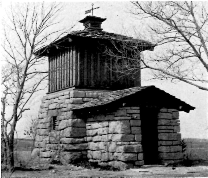
Pump House Bonham State Park Texas
