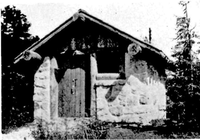
Pump House - - Wilderness State Park - - Michigan
