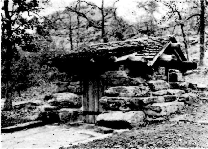
Pump House - Lake Murray State Park - Oklahoma
