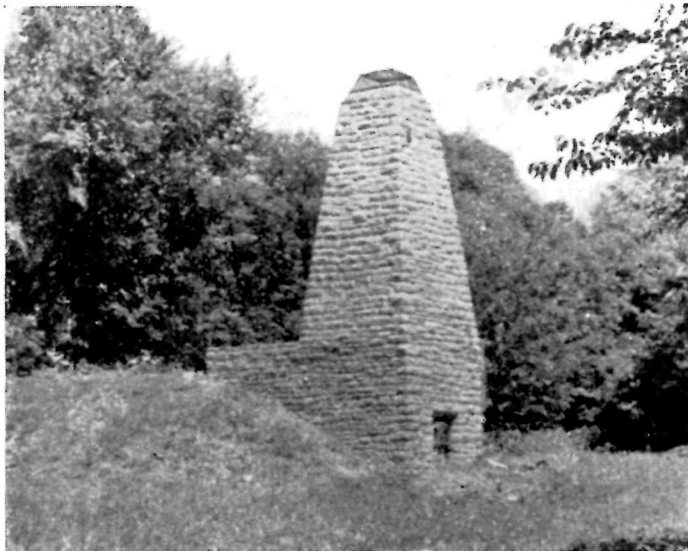
Incinerator, Sharon Woods, Cincinnati, Ohio
