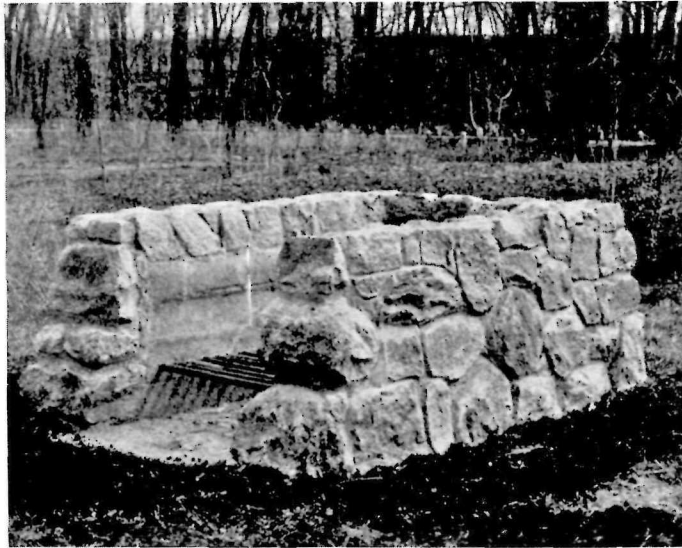
Incinerator, Fargo Metropolitan Park, North Dakota
