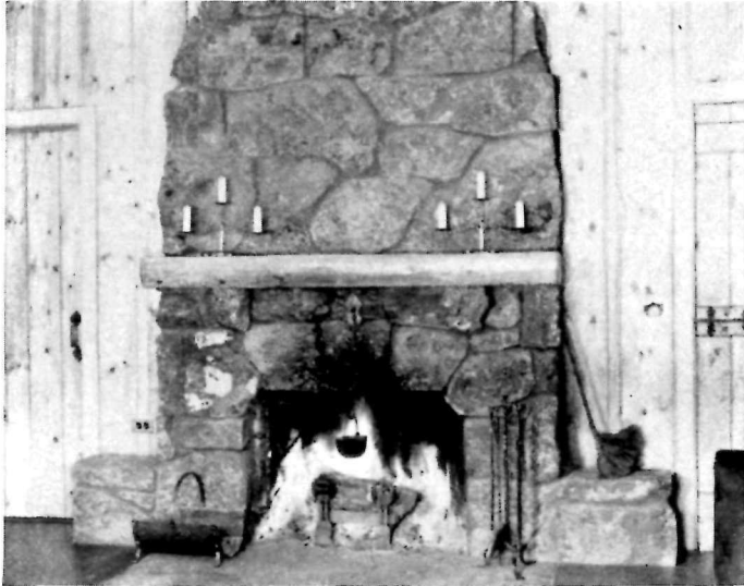
Caretaker's Dwelling, Riverside State Park, Washington
