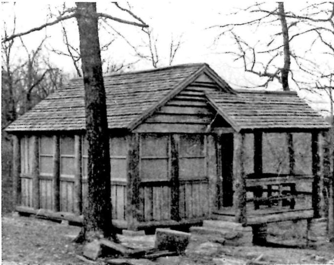
Falls Creek Falls Recreational Demonstration Area, Tennessee
