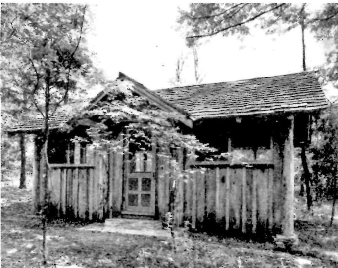
Otter Creek Recreational Demonstration Area, Kentucky
