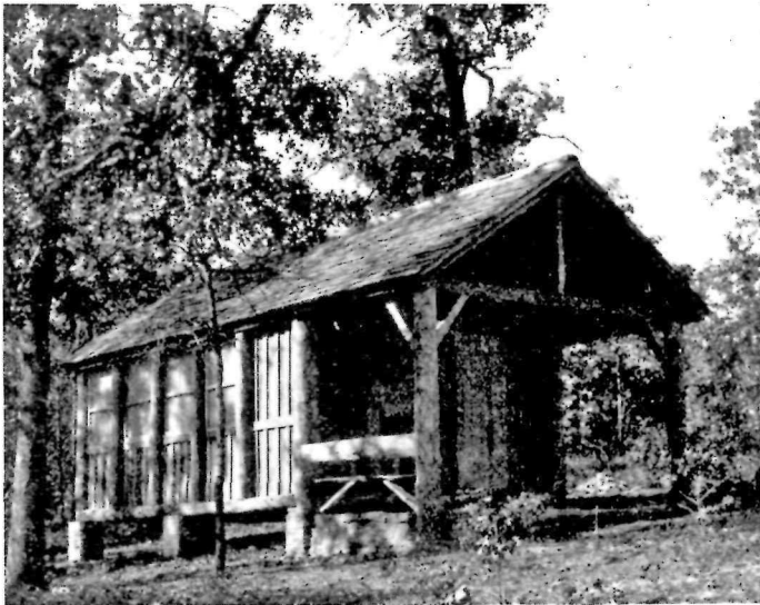
Falls Creek Falls Recreational Demonstration Area, Tennessee
