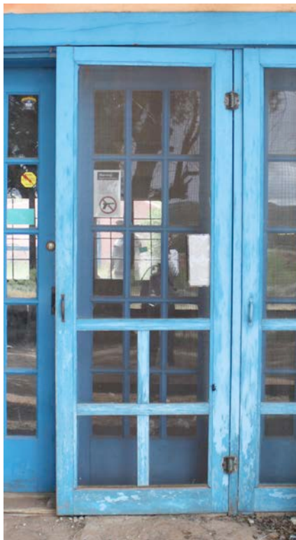
Exterior before treatment
