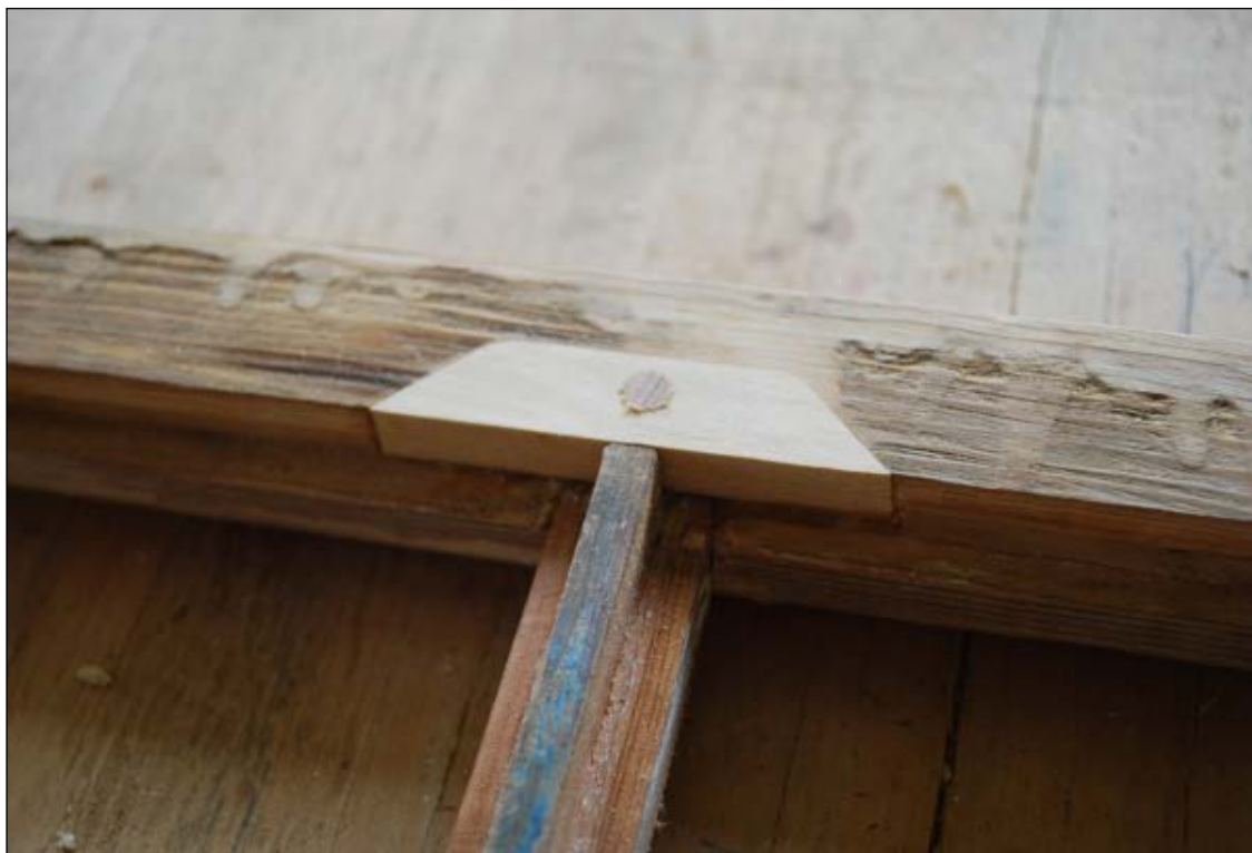
Figure 5. Dutchman repair at joint of meeting rail and muntin.
