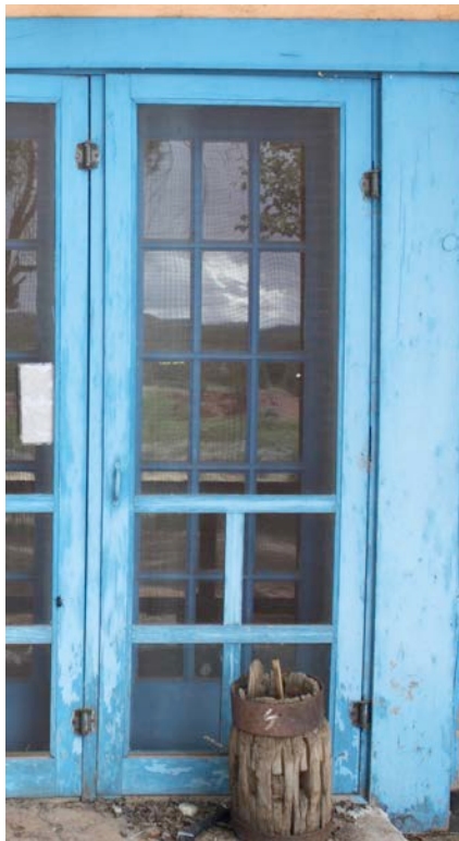
Exterior before treatment
