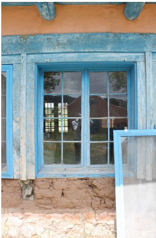
Exterior prior to treatment
