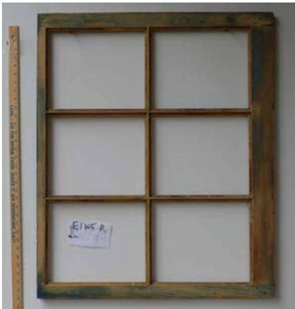
Right sash prior to treatment
