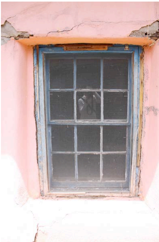
Exterior before treatment
