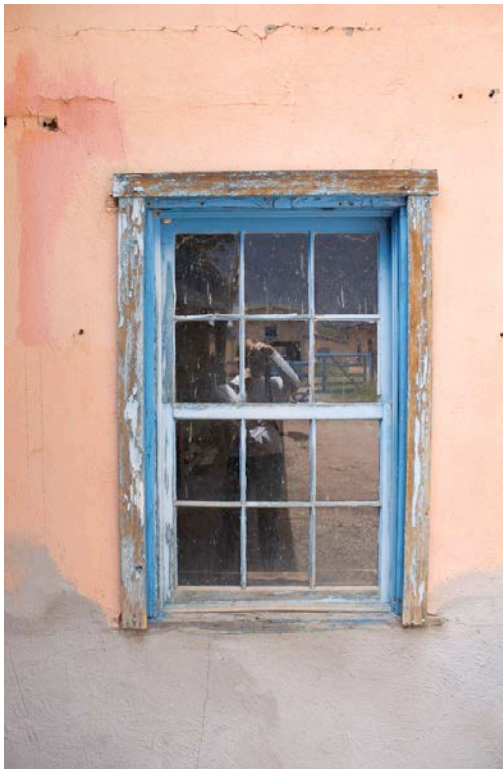
Exterior before treatment
