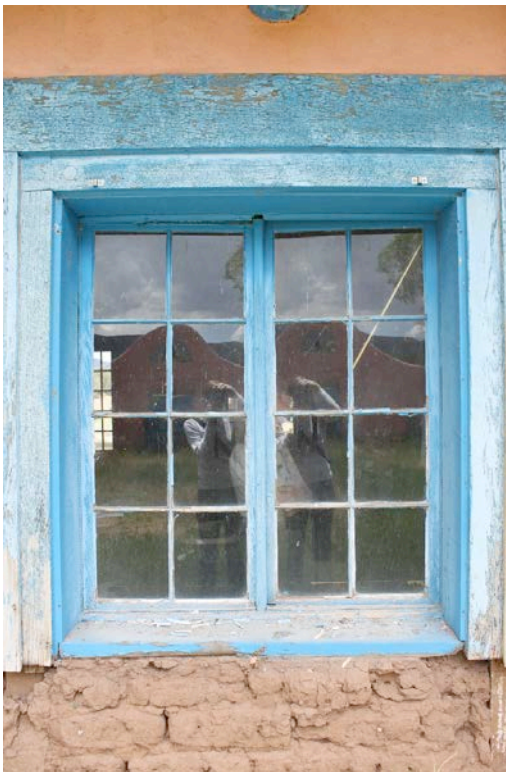
Exterior before treatment
