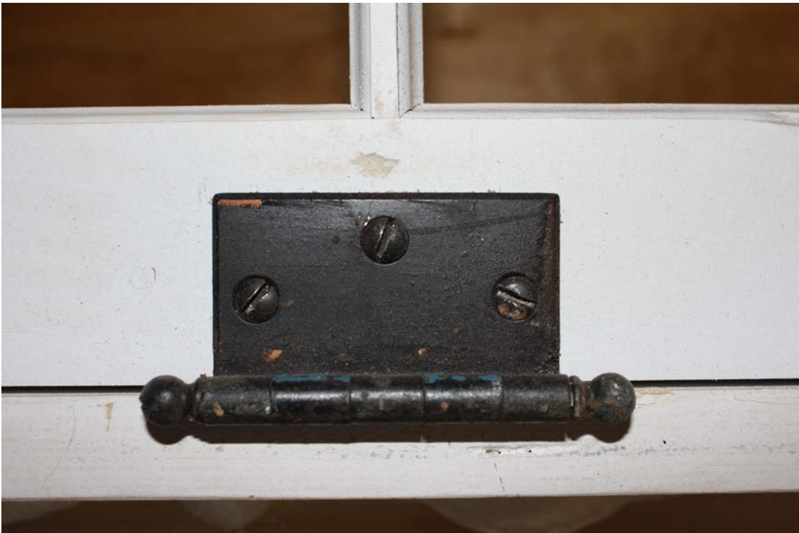
Figure 2. Casement window hinge
