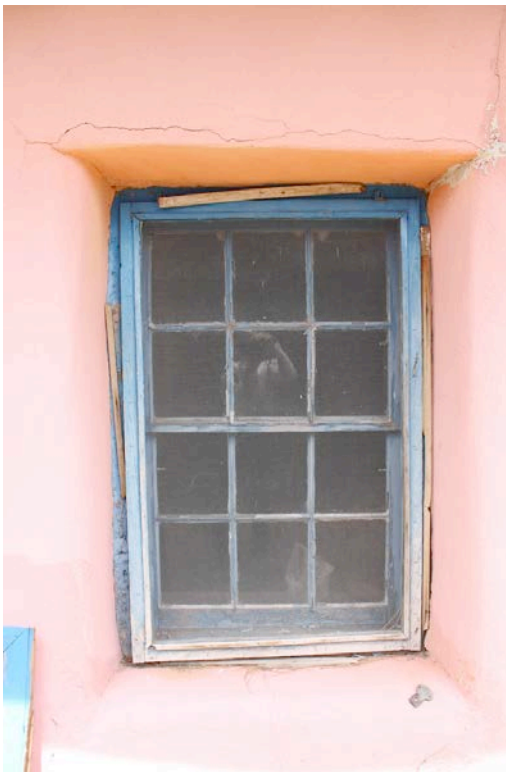
Exterior before treatment
