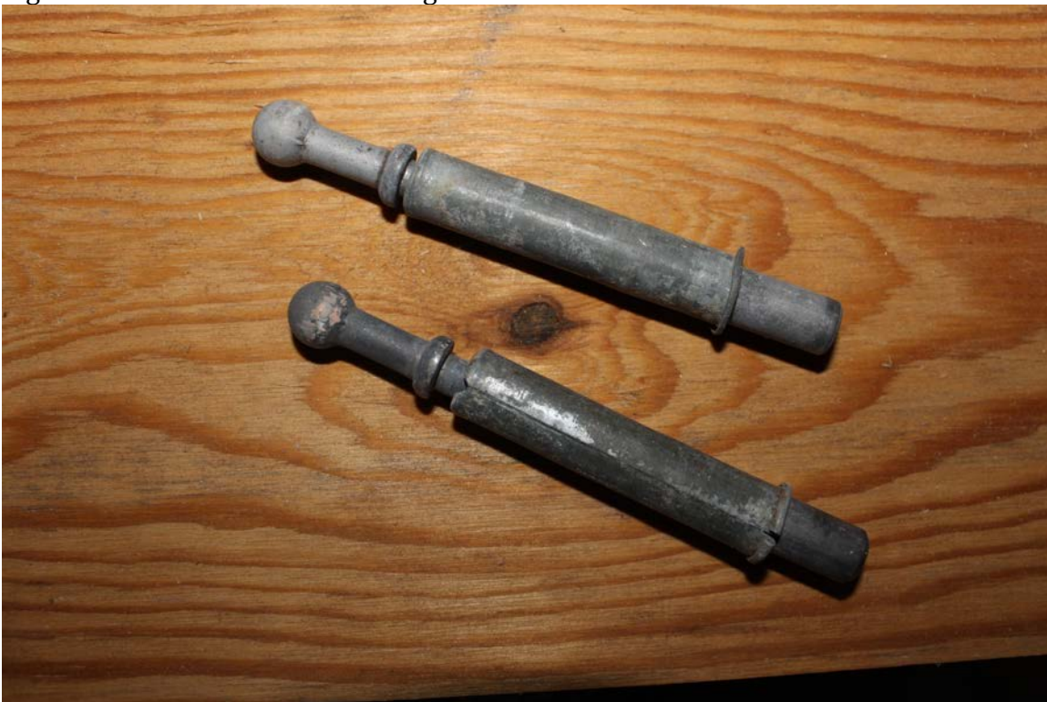
Figure 4. Sash bolts for sliding sash
