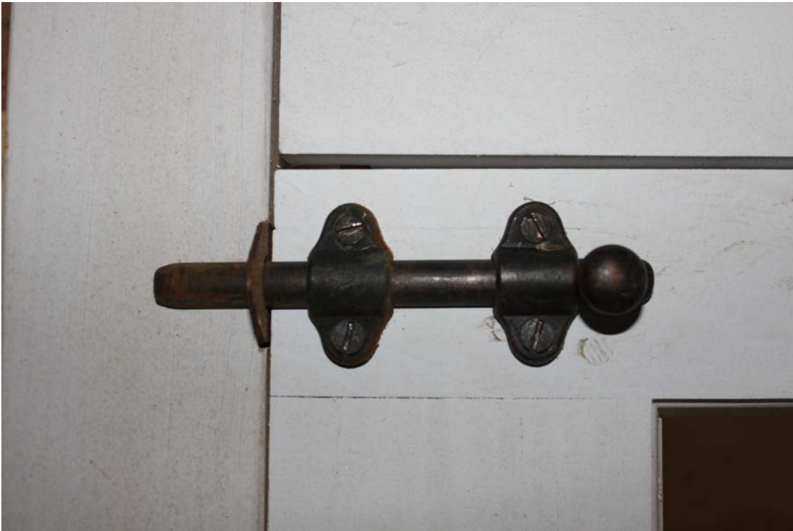
Figure 3. Casement window sliding surface latch bolt
