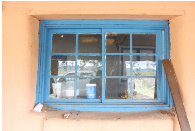
Exterior before treatment
