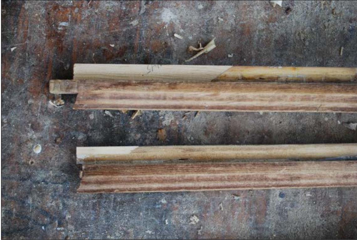
Figure 6. Repairs to damaged glazing bars on muntins.
