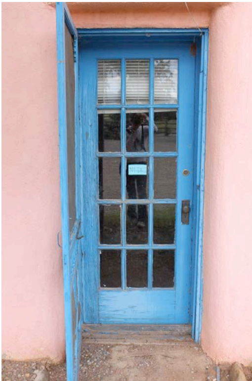
Exterior before treatment
