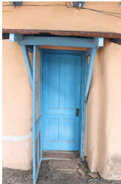
Exterior before treatment
