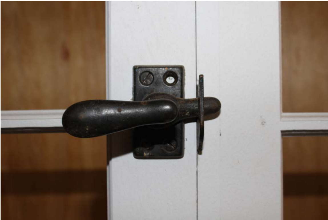
Figure 1. Casement window thumb latch and rim strike
