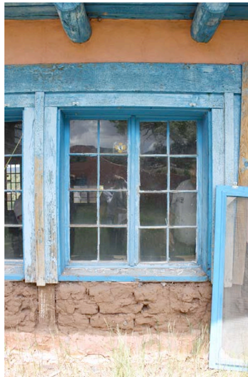
Exterior before treatment
