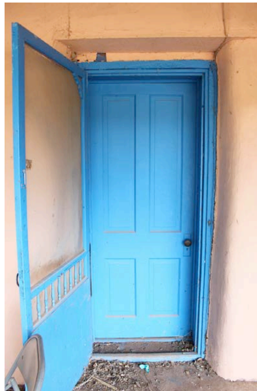
Exterior before treatment
