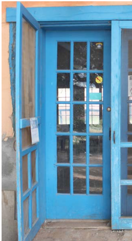
Exterior before treatment
