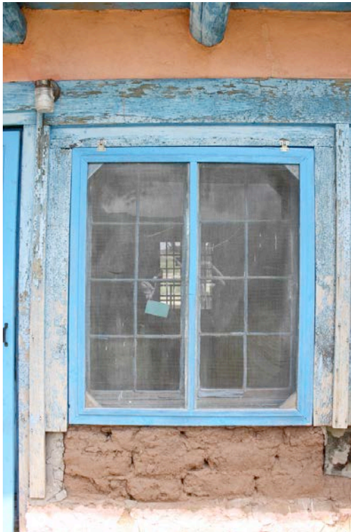
Exterior prior to treatment
