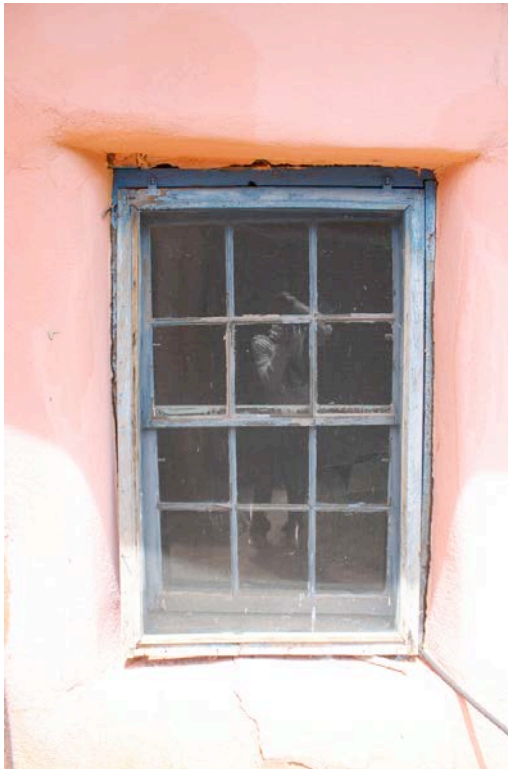
Exterior before treatment
