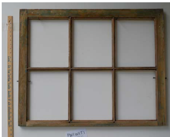
Upper sash prior to treatment
