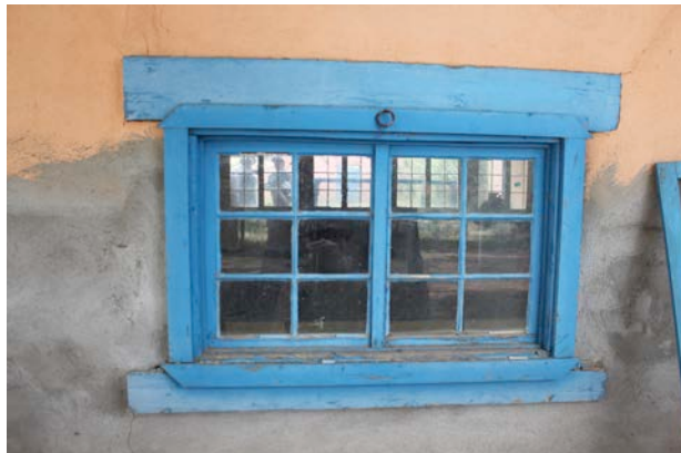
Exterior before treatment
