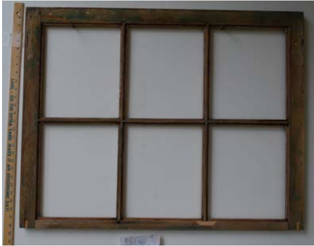
Upper sash after treatment
