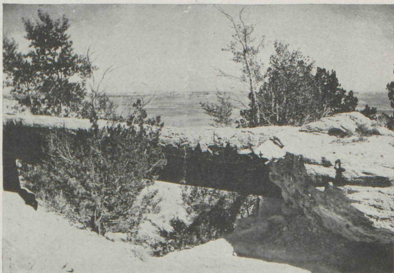
FIG. 7.—The Natural Bridge. Here the erosion of thousands of years has so exposed this log that its central portion spans an arroyo about 50 feet wide, while both ends still remain bedded in sandstone. Now strengthened by a reinforced concrete beam, seen in picture as a dark band under the log
