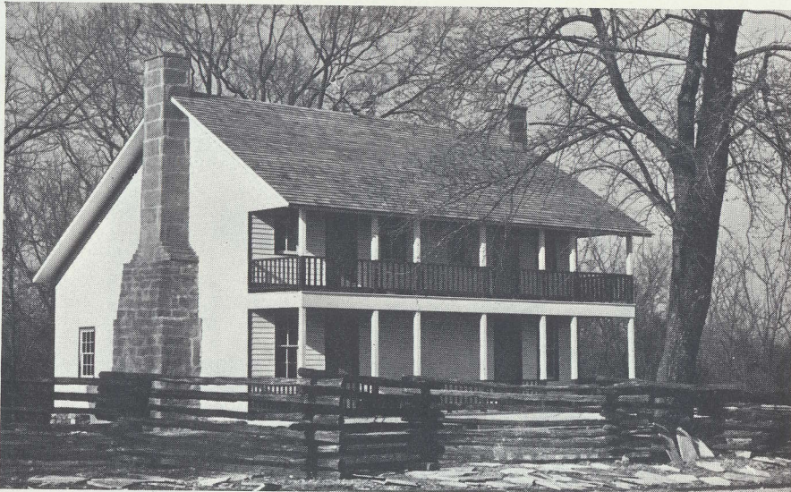
ELKHORN TAVERN —This restoration of the post-Civil War Elkhorn Tavern (the original was destroyed by fire about a year after the Battle of Pea Ridge) very closely resembles photographs of the building that date back as early as 1872. Elkhorn Tavern is now a historic house at Pea Ridge National Military Park.
