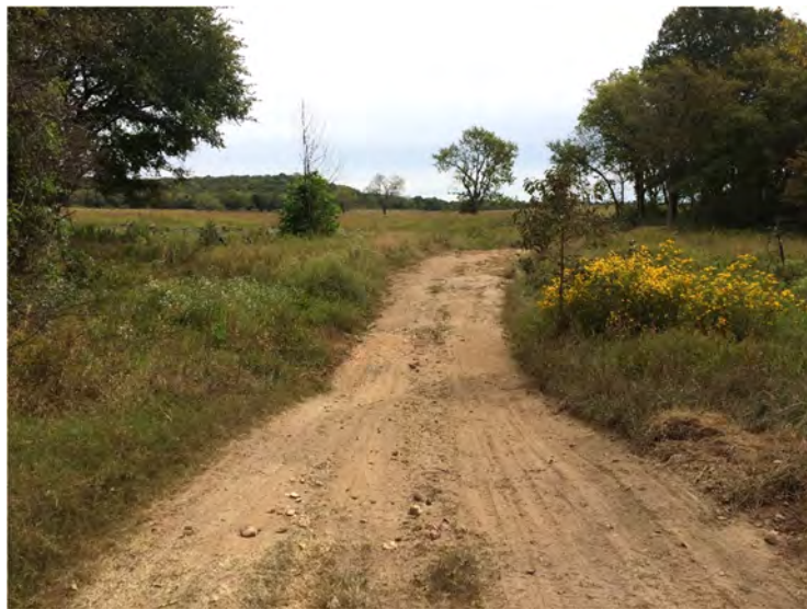
Figure 8. Ford Road Over Lee Creek Where Road Depression and Occasional Flooding Occurs
