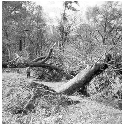
Damage to earthworks caused by windthrown trees.
