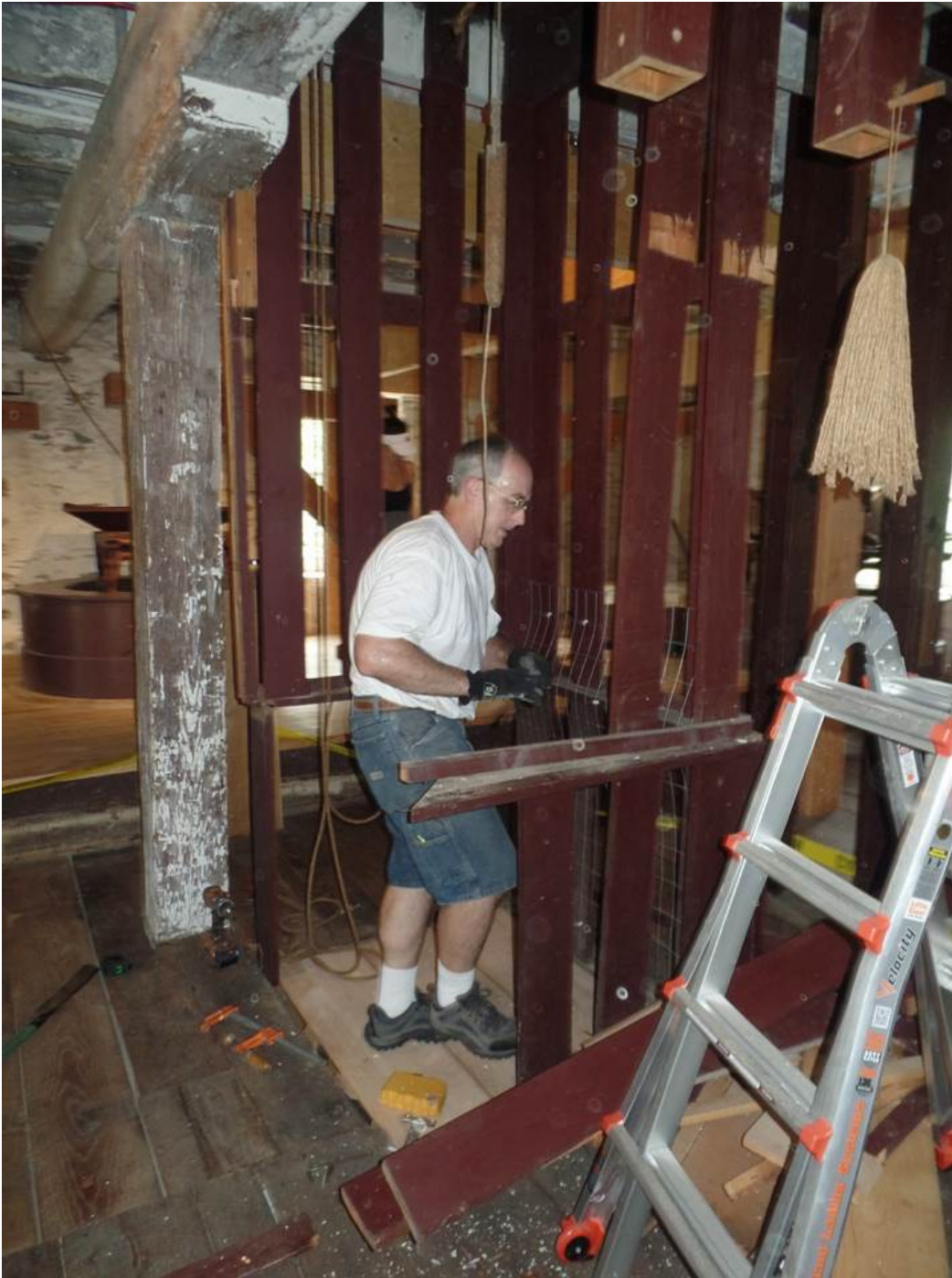
Mill restoration expert Steve Ortado removing the circa-1970s cage from the barrel hoist. (photo courtesy of Deborah Dougherty)
