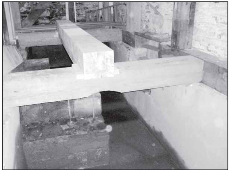
View of empty machinery pit and new stone bearer beam.
