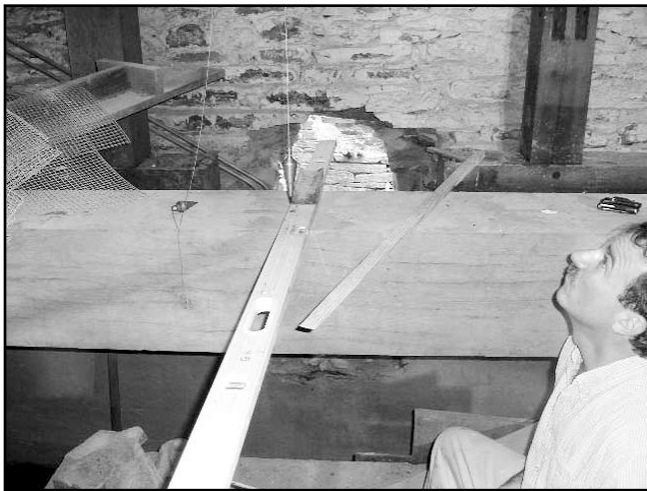
Gus Kiorpes takes measurements for the new main shaft
