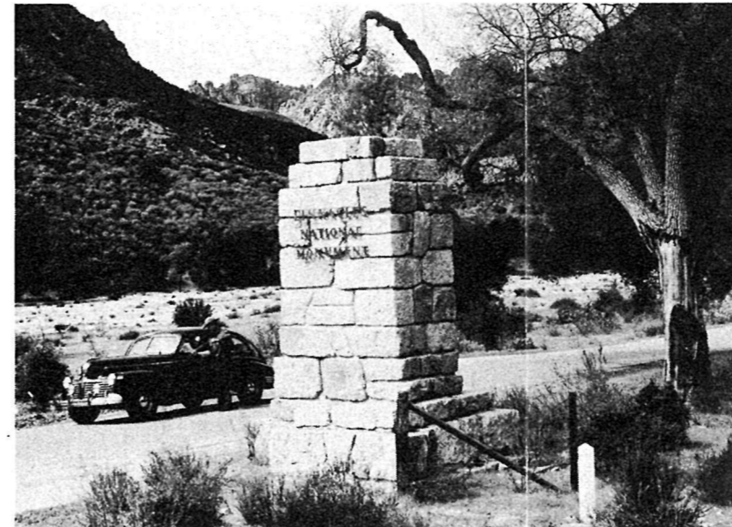
East entrance to Monument
