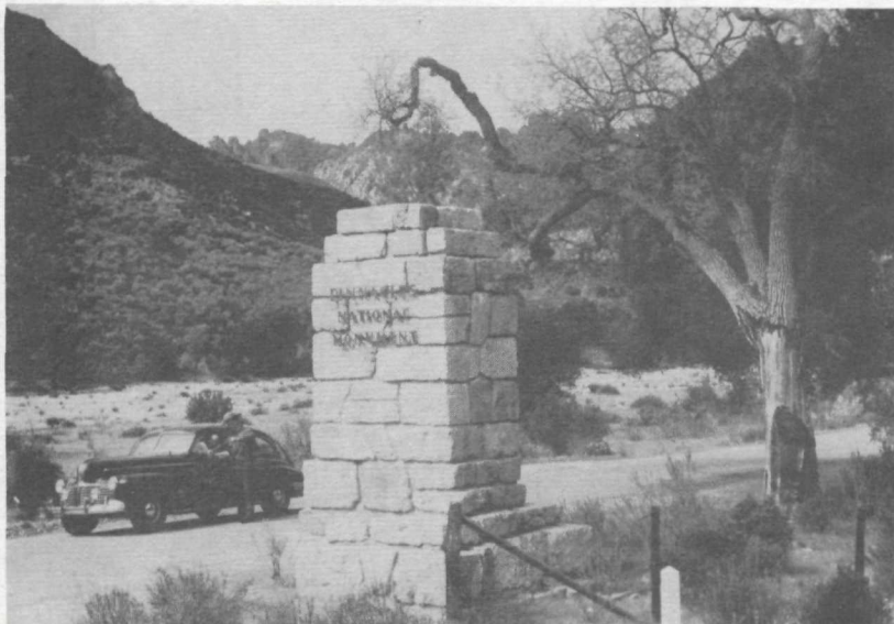
East entrance to monument
