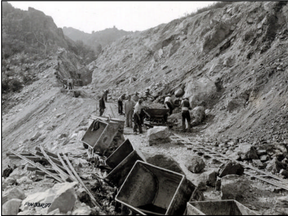
Figure 3 Construction of the Bear Gulch Road in the 1930s
