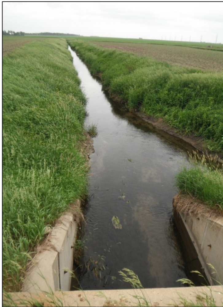
Figure 4-57. Upstream of the park, 13.9 miles of Pipestone Creek was channelized in the early 1900s turning the creek into a network of agricultural ditches. (CSU photo)
