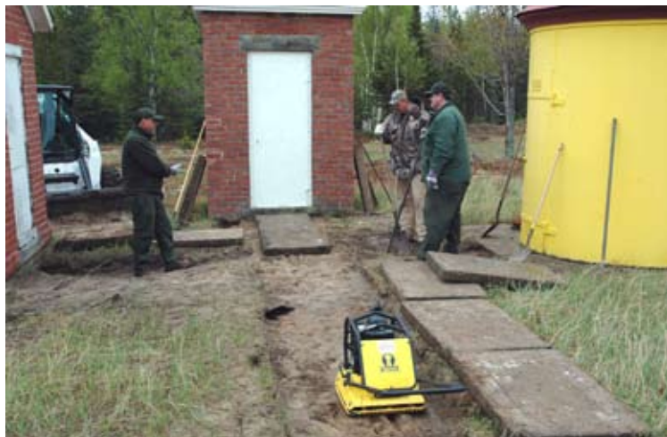
Sidewalk and landscape work
