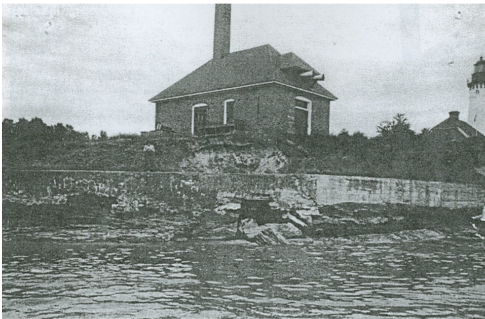
1950s photograph of fog signal building with deteriorated concrete seawall and 1942 extension (Louis Torres) (1999 CLR, p. 74). For full size image please reference the CLR Figure 32.
