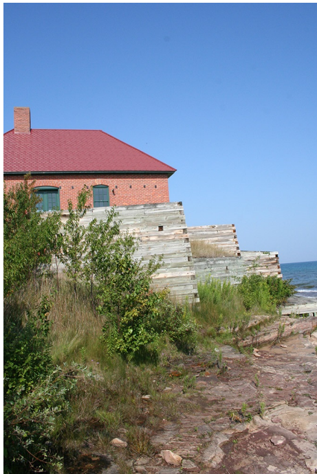
A human response to the natural environment is the continuous effort to shore up the sand bank. Note the log cribbing in the photo. (August 2012) Rusch/Young, NPS
