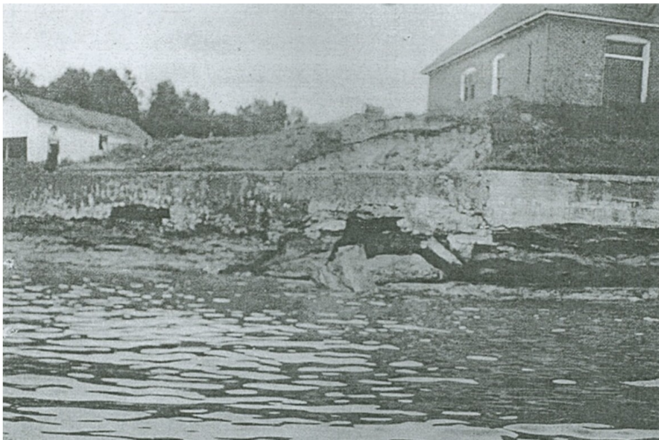
1950s photograph of deteriorated concrete seawall with boathouse and fog signal building (Louis Torres) (1999 CLR, p. 74). For full size image please reference the CLR Figure 31.
