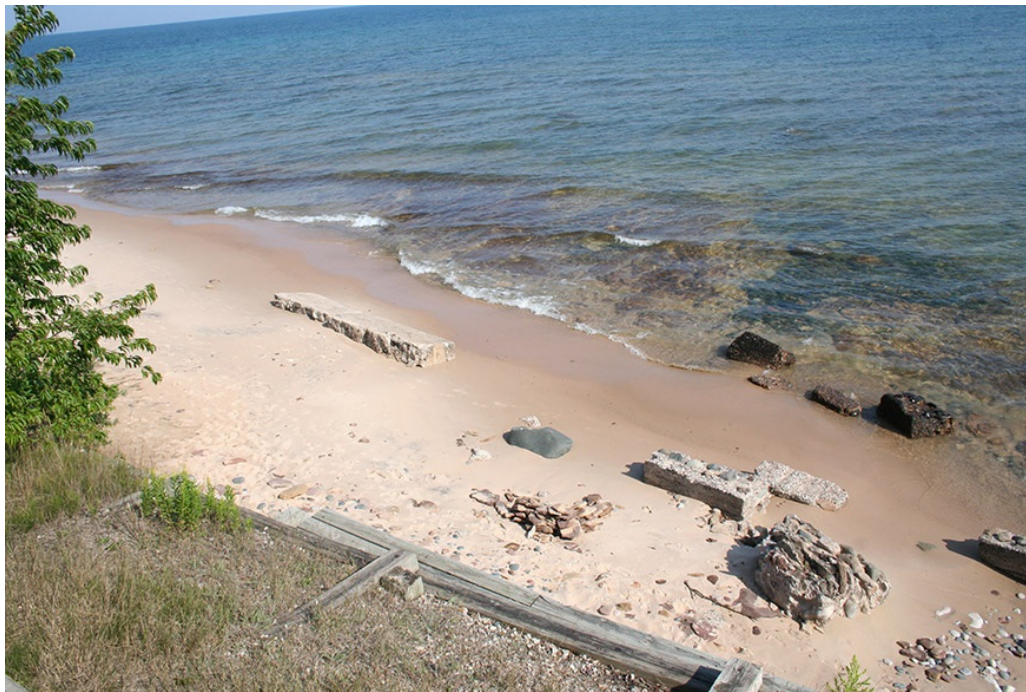
Concrete and wood remnants just below the modern wood cribbing stabilization effort along the shore. These remnants are indicative of the on-going effort to protect the site from erosion at this highly exposed site. (August 2012) Rusch/Young, NPS
