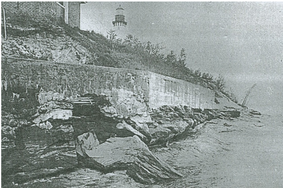
1950s photograph of shore protection at the fog signal building, showing 1942 seawall extension (Louis Torres) (1999 CLR, p. 73). For full size image please reference the CLR Figure 29.
