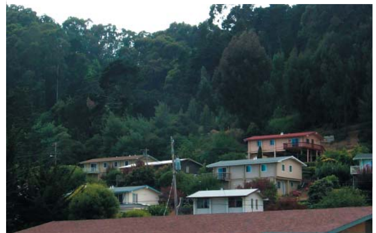
Below: Many homes in Marin City are surrounded by dense vegetation which is susceptible to wildfire.
