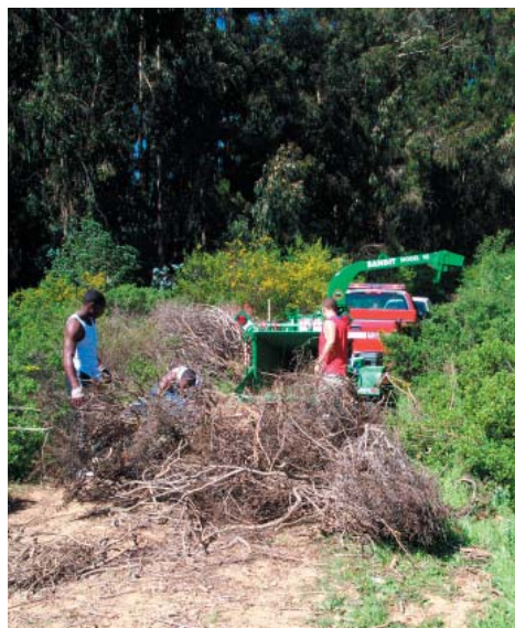
Marin County Fire Department assisted with the Alta Avenue project by providing the use of a chipper with supervision.
