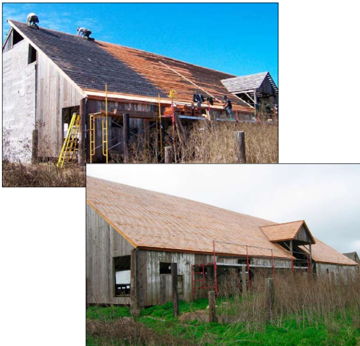
Stabilization of roof at the D Ranch Milking Barn
