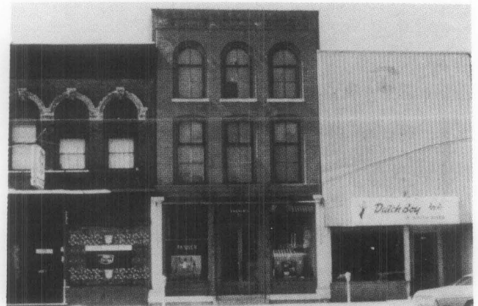
Figure 12. This photograph of three late 19th century commercial buildings clearly shows the impact of preserving and rehabilitating storefronts. The one on the right has been totally obscured by a "modern" front added in the 1950's. Although inappropriate alterations have taken place on the left storefront, it is still possible to determine the original configuration of the doors and display windows. The storefront in the middle has remained intact. Although in need of some minor maintenance work, the appeal of the original design and materials is immediately apparent.
