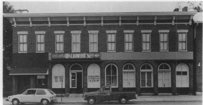
Figure 5. In some cases, as in the storefront on the extreme left, it is a simple matter to determine original appearance by looking at neighboring storefronts. Removal of the board and batten fasciabord, pent roof, and "colonial" style door, all of which could be undertaken at minimal cost, would restore the original proportions and lines of the building. Photo: Day Johnston
