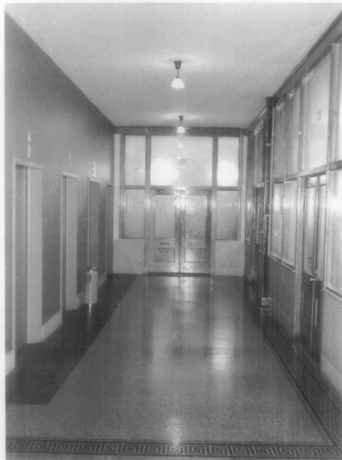
Figure 6. This corridor, located in the historic Monadnock Building in Chicago, has glazed walls, oak trim, and marble wainscoting, and is typical of those found in late 19th and early 20th century office buildings. Despite the simplicity of the features, a careful attention to detail can be noted in the patterned tile floor, bronze mail chute, and door hardware. The retention of corridors like this one should be a priority in rehabilitation projects involving commercial buildings.
