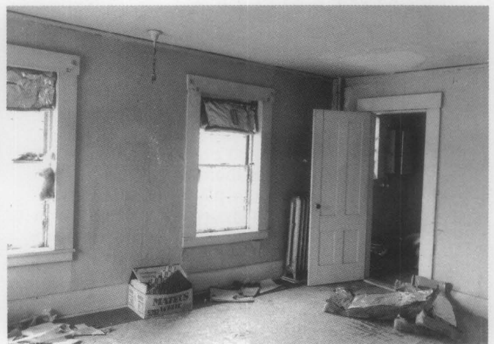
Figure 5. The interior of a simply detailed worker's house of the 19th century may be as important historically as the richly ornamented interior seen in figure 1. Although the interior of this house has not been properly maintained, the wide baseboards, flat window trim, and four-panel door are characteristic of workers' housing during this period and deserve retention during rehabilitation.
