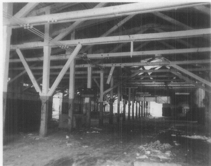
Figure 2. The interiors of mills and industrial buildings frequently are open, unadorned spaces with exposed structural elements. While the new uses to which this space could be put are many—retail, residential, or office—the generous floor-to-ceiling height and exposed truss system are important character-defining features and should be retained in the process of rehabilitation.
