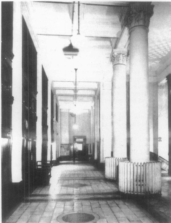
Figure 9. The tangible reminders of early mechanical systems can be worth saving. In this example, in the Old Post Office in Washington, D.C., radiators encircle Corinthian columns in a decorative manner. Note, too, the period light fixtures. These features were retained when the building was rehabilitated as retail and office space. Photo: Historic American Buildings Survey
