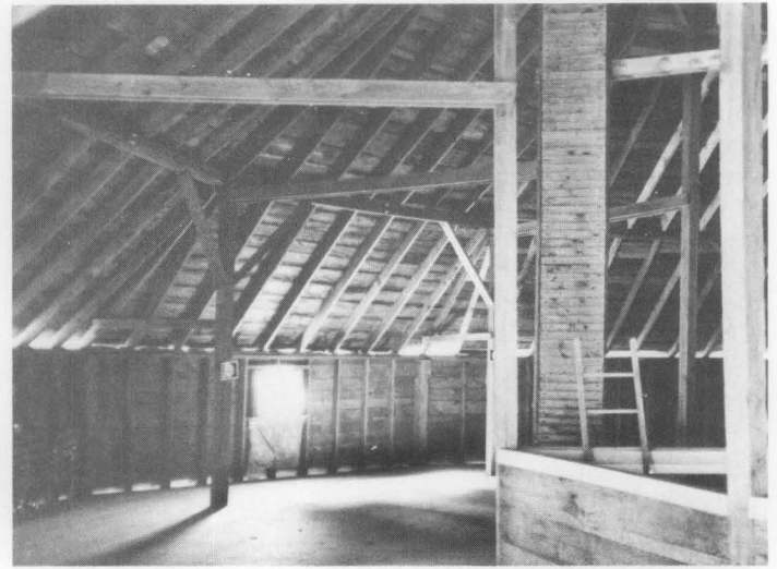
Fig. 10. This 1910 Vermont round barn is 80 feet in diameter. Disused and decaying, the building was converted to a community center, with artists' studios and spaces for weddings, parties and conferences. The barn underwent extensive structural repair and other work. Careful selection of new use permitted the building to be rehabilitated while retaining its principal spaces and features—and its historic character—intact. Photos: Jay White.
