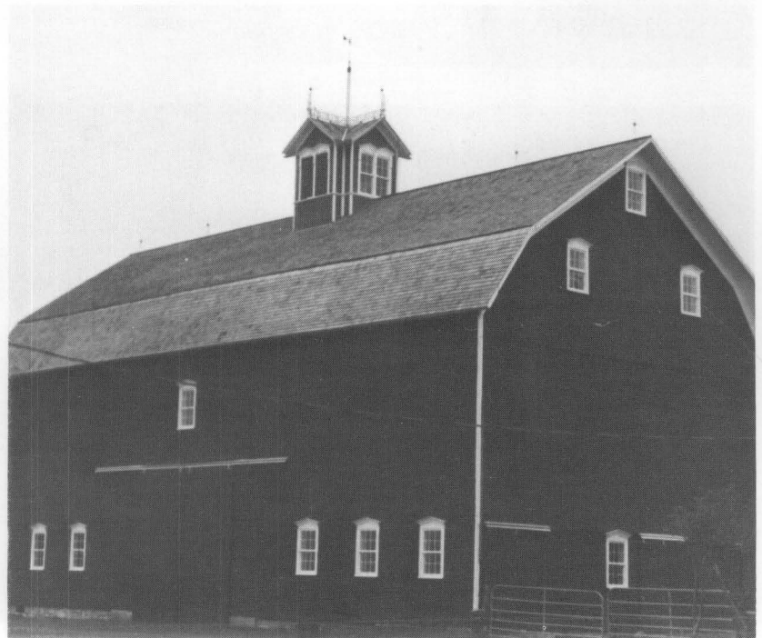
Fig. 8. Built in the Gothic Revival style in the 1890s, this four-story Indiana barn had fallen into disuse, and was deteriorating. In the process of returning it to use, the owner installed a new roof that matches the wooden shingles found beneath the deteriorating asphalt shingle roof; removed the modern asbestos shingle siding; repaired the windows, and reconstructed the cupola (including its lightning rod and weathervane). (Before and after views are of opposite sides of barn.) Photos: Before, Courtesy, Gary Post-Tribune; After, Courtesy, Kankakee Valley News.
