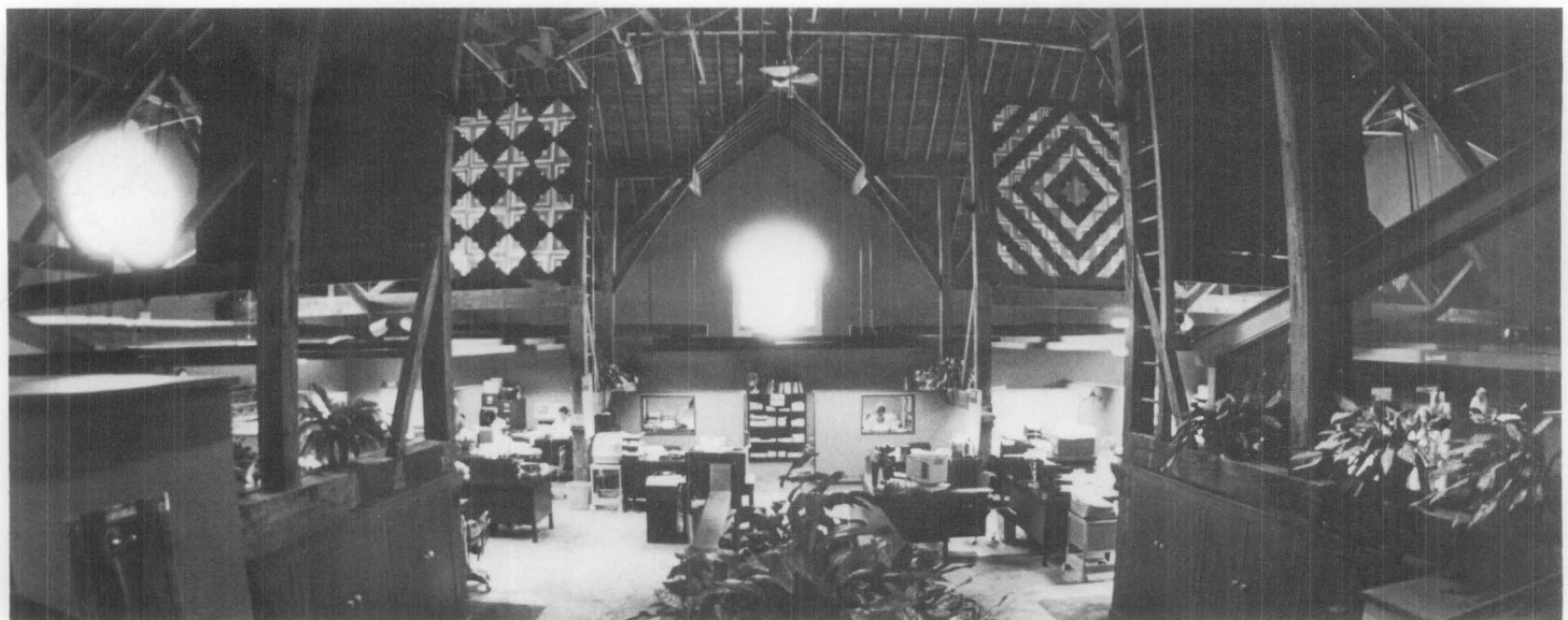
Fig. 9. This enormous Ohio barn (285 feet by 125) was built between 1909 and 1912. It was one of 102 structures on "America's Finest Farm." (Other buildings included the world's largest greenhouse and the world's largest barn—nearly 800 feet long). The barn seen here was rehabilitated for use as headquarters for an international agricultural firm. Although the use has changed, comparison of the interior photographs shows that the barn has retained its historic character. (After view, interior, is taken from a cross axis; distortion is from fish-eye lens.) Photos: Exterior and interior, after: Ron Kuntz, UPI; Interior, before: Courtesy, Barberton (Ohio) Historical Society.
