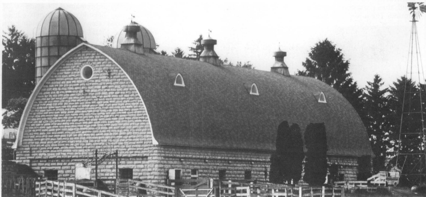
Fig. 1. Arch roof, native limestone walls two feet thick at the base, porthole window, dormers, silos, rooftop ventilators, weathervanes, windmill, fences, fields, and family pride in the builder are all components of the historic character of this Iowa barn. Photo: John Walter, Successful Farming.
