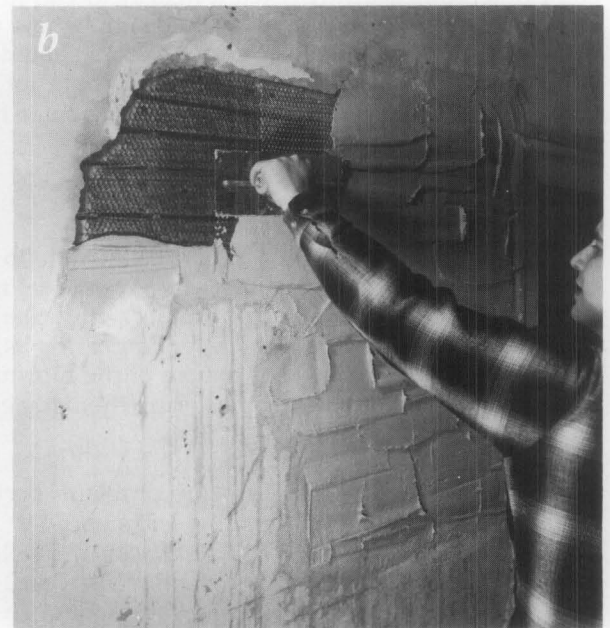
Fig. 10 (a) and (b). In this New Hampshire residence dating from the 1790s, the original plaster was a single coat of lime, sand, and horsehair applied over split lath. A one-coat repair, in this case, is appropriate. To the left: a flat sheet of galvanized expanded metal lath is placed over the patch area and an outline marked with a large soft lumber crayon. The metal lath is then cut to fit the hole and nailed to the lath. To the right: the edges of the original plaster and wood lath beneath have been thoroughly soaked with water. A steel trowel is used to apply the plaster in large, rough strokes. Finally, it will be scraped and smoothed off. Because only one coat of plaster is used, without a finish coat, a clean butt-joint is made with the original plaster. Photos: John Leeke.
