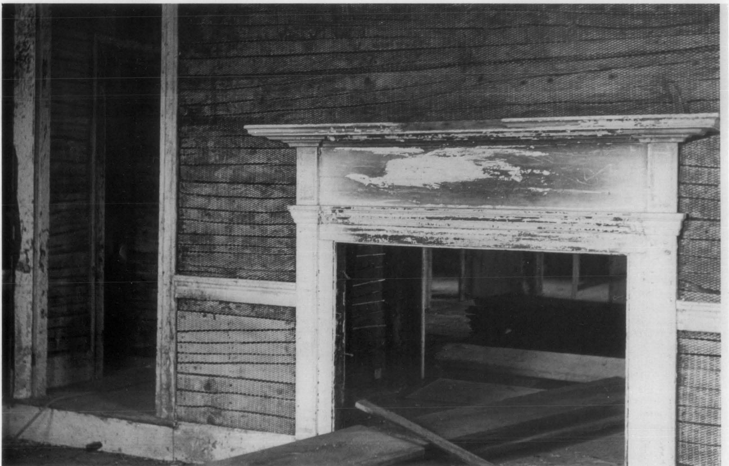
Fig. 16. In the restoration of a ca. 1830s house in Maine, split-board lath has been covered with expanded metal lath in preparation for new coats of plaster. This method permits the early lath to be saved while the metal lath, with its superior keying, serves as reinforcement. Photo: National Park Service files.
