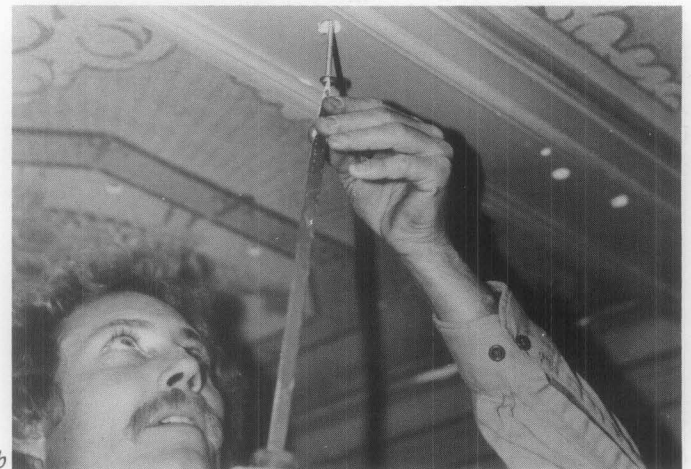
Fig. 17 (a) Where this ceiling was suffering from structural failure, the first step was to shore it up from below. (b) Toggle bolts were used to reattach the plaster molding to the ceiling joists. The ceiling was then patched with gypsum and lime, prior to restoring the significant paint finishes. Photos: National Park Service files.
