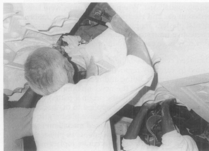
Fig. 23. A pre-cast coffer is lifted into place to abut adjacent panels. Tie wire will be fastened to the channel irons and the superstructure above, twisted to level, and finally wadded with wood fiber soaked in plaster to prevent the wire from stretching. Photo: David Flaharty.
