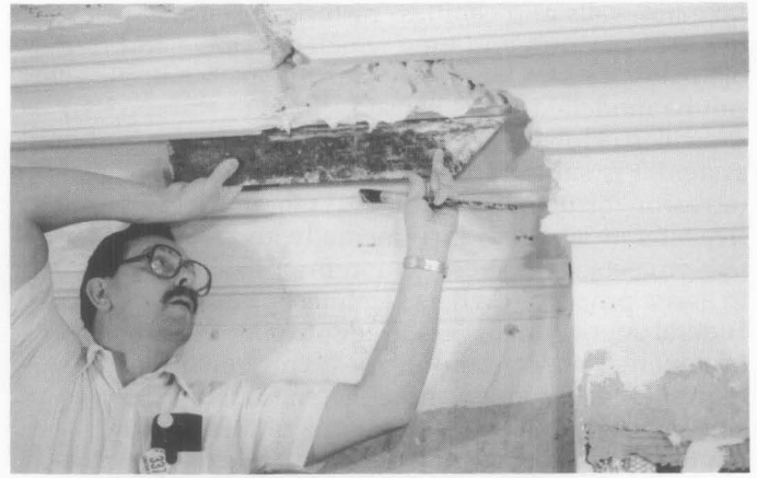
Fig. 5. Mitering a Plain-Run Cornice. Mitering requires great dexterity using the miter rod. In this case, a return at a chimney breast is tooled using an infill of gypsum and lime. Internal and external miters are required with the internal being the most difficult. Another method is to run a length of cornice (using the same blade) on a bench and set it in place, later to point the joints. Photo: Old-House Journal.
