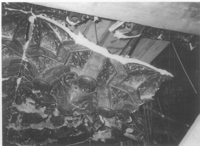
Fig. 21. The Yiddish Arts Theater, New York City, c. 1920s. The concrete roof of this building collapsed, damaging portions of the existing Moorish style coffered ceiling. The square coffer unit was easily identifiable and was removed to a casting shop for reproduction. Photo: David Flaharty.
