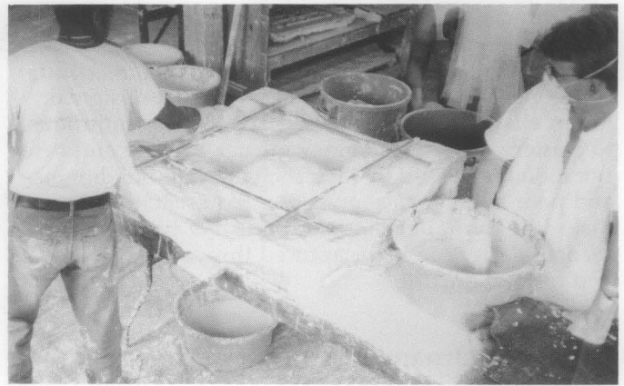
Fig. 8. Casting a Coffering Unit. Ceiling coffers are made the same way today except, historically, a hide glue mold was poured over an ornamental model whereas today urethane molding rubber is used. Now, as then, the plaster casts are made with steel channel irons embedded on the back of each panel. The coffers are hung from carrying irons fixed to the ceiling above by means of twisting wires to level each coffer to its neighbor. Afterward, the panels are fastened together and the joints pointed with plaster. Photo: David Flaharty.
