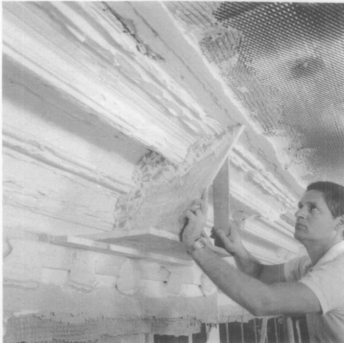
Fig. 4. Running a Cornice. The historic method of producing a cornice is unchanged today. A running mold or template is pushed along a lattice strip nailed to the wall. Base coat plaster is gypsum and sand; finishing plaster is added with small tools and stuffed wearing rubber gloves because lime burns the skin. As many as 20 passes are required to complete a smooth run; this particular cornice was formed in two stages, top and bottom, because it was so large. Cornices this size also have to be blocked and lathed to minimize the amount of applied material. Photo: Old-House Journal.
