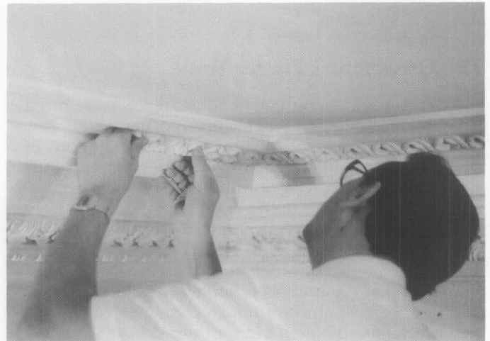
Fig. 6. Enriching a Plain-Run Cornice. After a cornice is run and mitered, cast enrichments are stuck in recessed sinkages planned to receive the casts. Ornamental models are made to engage with one another, resulting in unbroken lines or courses. A shop-cast ornament is soaked in water until saturated and pressed into its sinkage using wet plaster as an adhesive. Once the casts have been installed, they are carefully pointed at the joints and at the miters so that they appear as a continuous, repetitive design. Photo: Old-House Journal.
