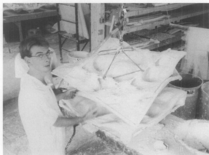
Fig. 22. Repairing a Coffered Ceiling. As part of the theater rehabilitation, the coffered ceiling panels are being reproduced in urethane rubber molds and reinforced with open weave burlap and wood fiber. Steel channel irons can be seen, attached to the backs of the casts. Later, these irons are used to hang the panels from a superstructure at the site. Photo: David Flaharty.
