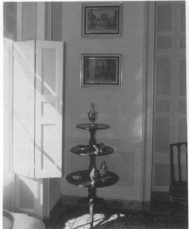
f. Homewood, Baltimore, MD. This elegant circa 1806 residence is now a house museum. The registers for the forced air ducted system seen behind the table legs, are grained to blend with the historic baseboards. The HVAC system uses a water/air system where chilled water and steam heat are converted to conditioned air. Photo: Courtesy Homewood Museum, Johns Hopkins University.
