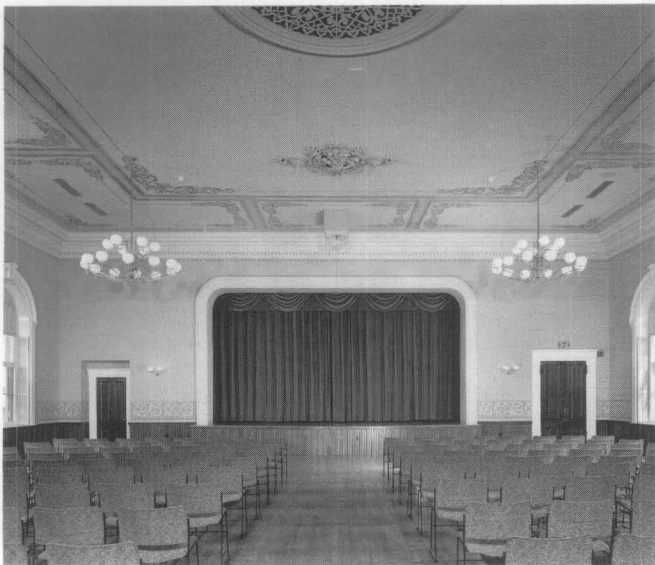
e. Town Hall, Andover, MA. The upstairs auditorium was restored and new mechanical systems were installed. Perimeter baseboard radiation provides heat and air handlers, located in the attic space provide air conditioning. The cast iron ceiling grille was adapted for return air and the supply registers were installed in a symmetrical and regular manner to minimize impact on the historic ceiling. Photo: David Hewitt/Anne Garrison for Ann Beha Associates.
