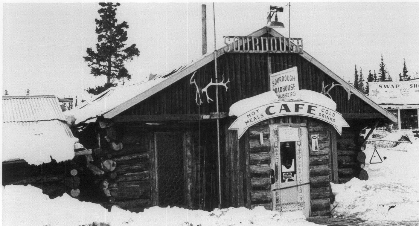
Fig. 1. Log construction was practical in the rough frontier and climate of Alaska, where it was used for a variety of structures such as the Sourdough Lodge (c. 1903) near Gakona. Built to serve the trail leading to the Klondike gold discoveries, this 1-story, L-shaped roadhouse is primarily of horizontal log construction with vertical logs in the front gable. Photo: National Park Service Files.
