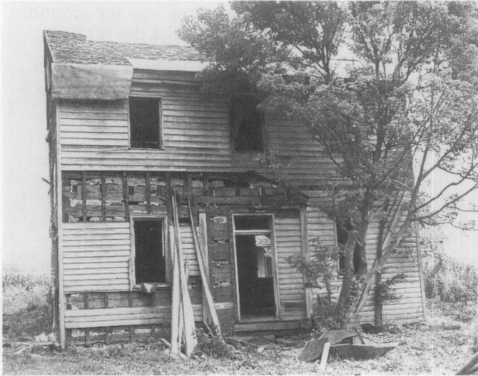
Fig. 14. Removal of the historic wood siding from the 1804 Zachariah Price DeWitt House in Butler County, Ohio, reveals that the clapboards were attached to vertical wood furring strips nailed to the logs. Photo: National Park Service Files.
