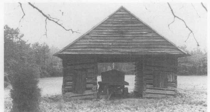
Fig. 3. This mid-19th century double-pen corncrib on the Jamison Farm in Rowan County, North Carolina, is an example of a type of log building that did not require chinking. Photo: Denise Whitley.
