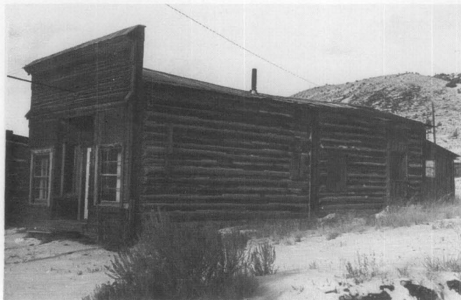
Fig. 4. Beginning around the mid-19th century, entire western boomtowns were hastily constructed of frame and log, such as the buildings in Bannack, Montana, the site of the State's first gold discovery. Photo: National Park Service Files.
