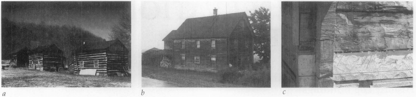
Fig. 2. Logs, both round and hewn, continued to be a basic construction material throughout much of the 19th century, here illustrated by (a) these c. 1831 industrial workers' houses for forgersmen at the Mt. Etna Iron Furnace in Pennsylvania, and (b) the Larsson-Ostlund House built by Swedish immigrants in New Sweden, Maine, during the 1870s. (c) Corner detail of the Larsson-Ostlund House with the original clapboarding removed during restoration shows close-fitting log joints in the Scandinavian style that did not require chinking. Photos: (a) Jet Lowe, HAER Collection, (b-c) Maine Historic Preservation Commission.
