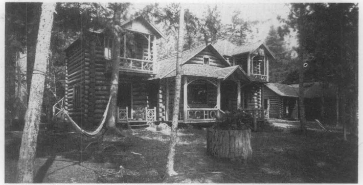
Fig. 5. The main lodge of Echo Camp on Raquette Lake in New York State was built in 1883 by the governor of Connecticut. It typifies the Adirondack style in the use of exposed round logs with crowns, and porches and balconies constructed with bowed logs and round log columns. Photo: Courtesy The Adirondack Museum.
