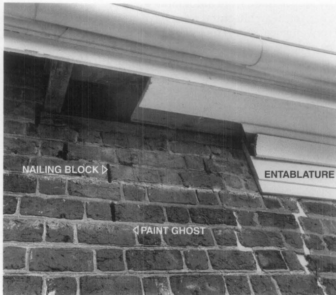
Figure A. Careful examination of the masonry reveals different periods of construction and repair through the composition and detailing of bricks and mortar. Depending upon location, open vertical joints may indicate the location of nailing blocks for decorative trim or weeps for drainage. These open joints at the building's cornice show evidence of an earlier wooden entablature extending down two courses below the present trim. The paint ghosts below the lowest blocks confirms the entablature's existence and provides clues to its size and finish.
