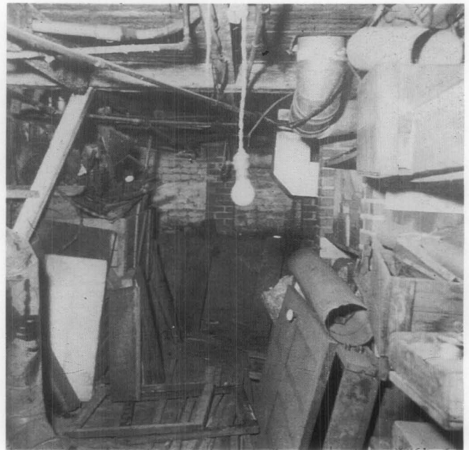
Figure F. Outdated fixtures and systems are frequently abandoned in place when more modern units are installed. Examining and documenting their existence can provide a technological reference to the history and use of many rooms or structures. photo: NPS Preservation Assistance Division Files.
