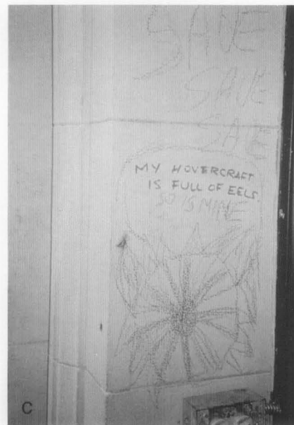
Figure 3 (a-d). A wide variety of materials is used to make surface-applied graffiti on masonry, including (a) chalk, (b) felt-tip marker, (c) felt-tip marker combined with crayon, and (d) felt-tip marker and spray paint on concrete. Photos: (a) Anne Grimmer, (b) Frances Gale, (c) Martin Weaver, (d) Anne Grimmer.
