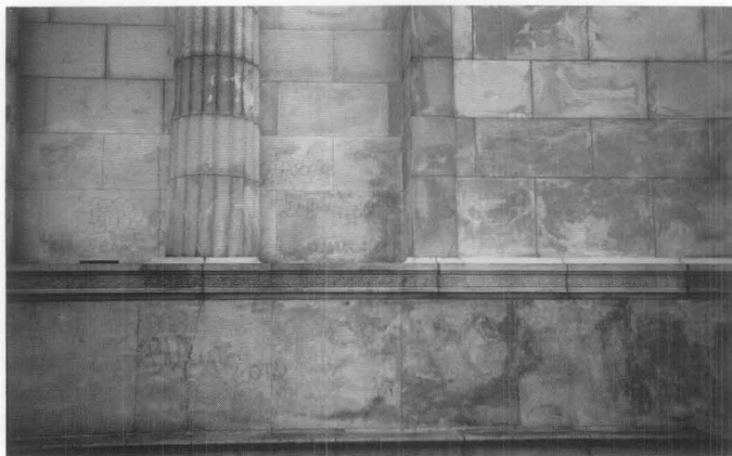
Figure 2. Harsh, but ineffective, graffiti removal methods have resulted in permanent damage to granite walls at the General Grant National Memorial in New York City. Photo: Judith M. Jacob
