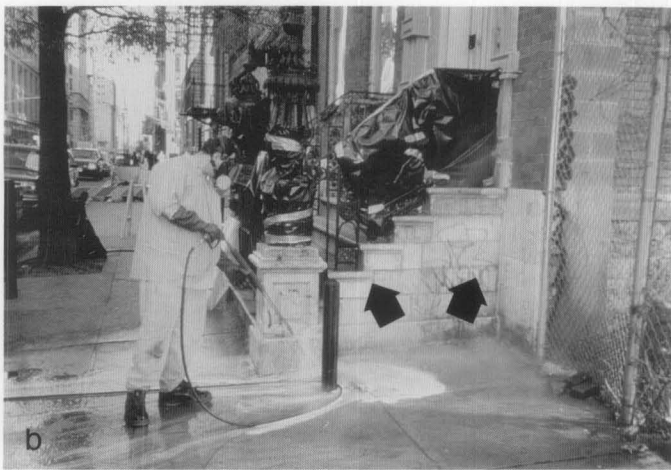
Figure 4 (a-b). After cleaning with an alkaline paint remover, remnants or ghosts of black spray-painted graffiti are still visible and may require poulticing, while the blue paint has been almost completely removed. Photos: Mark A. Weber.
