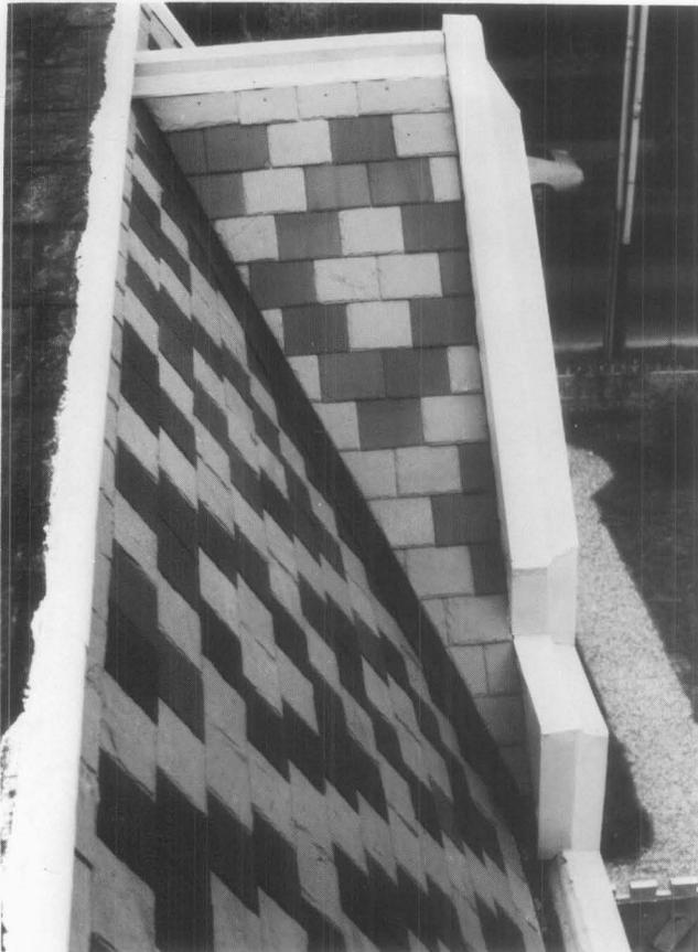
*The Victorians loved to use different colored slates to create decorative patterns on their roofs, an effect which cannot be easily duplicated by substitute materials. Before any repair work on a roof such as this, the slate sizes, colors, and position of the patterning should be carefully recorded to assure proper replacement. (Ebenezer Maxwell Mansion, Philadelphia, Pennsylvania, photo courtesy of William D. Hershey)*
